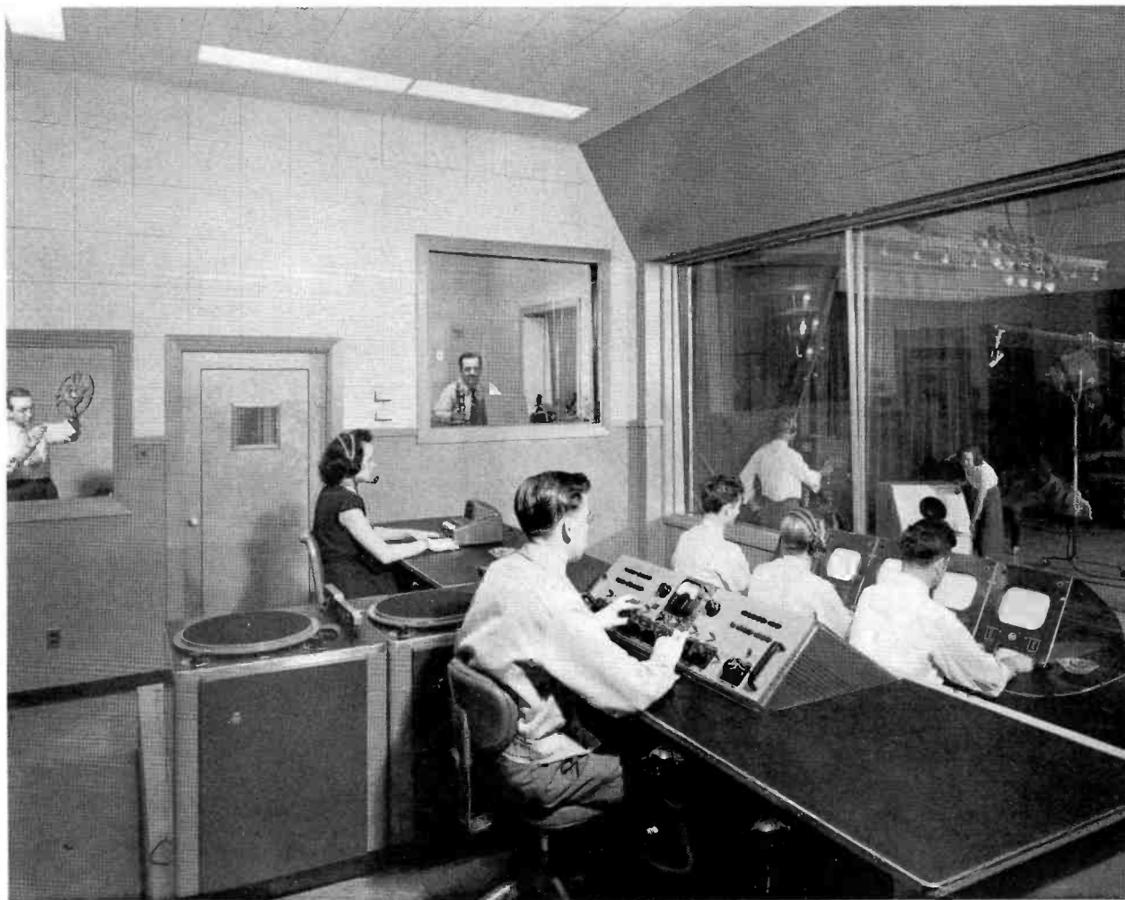
FIG. 8 (below). The announcer's booth at WHIO's new television station is surrounded on three sides by the studio control room (foreground), the studio proper (which is seen through the control room window on the right), and the projection room (through window on left), so that the announcer can see what is going on at any time in all three places. Speakers have been concealed behind flush-perforated panels above the window. The ceiling and upper walls are natural color fiber acoustic tile. The lower walls are plaster painted blue-gray.
