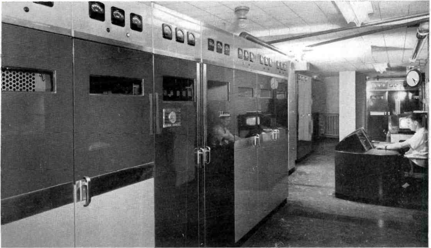
FIG. 11. WTCN's television transmitter, TT-5A at left, and the 3 KW FM transmitter in background at right, are located on the 28th floor of the Foshay Building. Mr. Bert Coil, Transmitter Supervisor, is at the transmitter control console.
