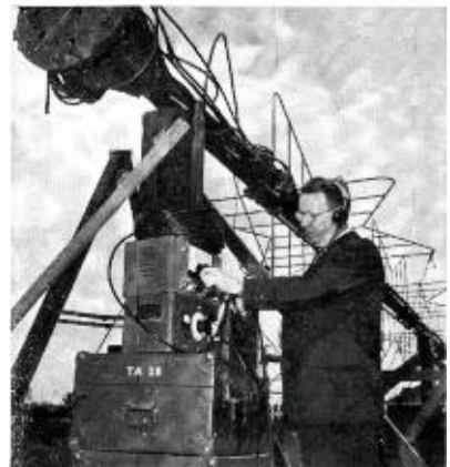
Ground-checking a 3-bay TV Super-Turnstile
