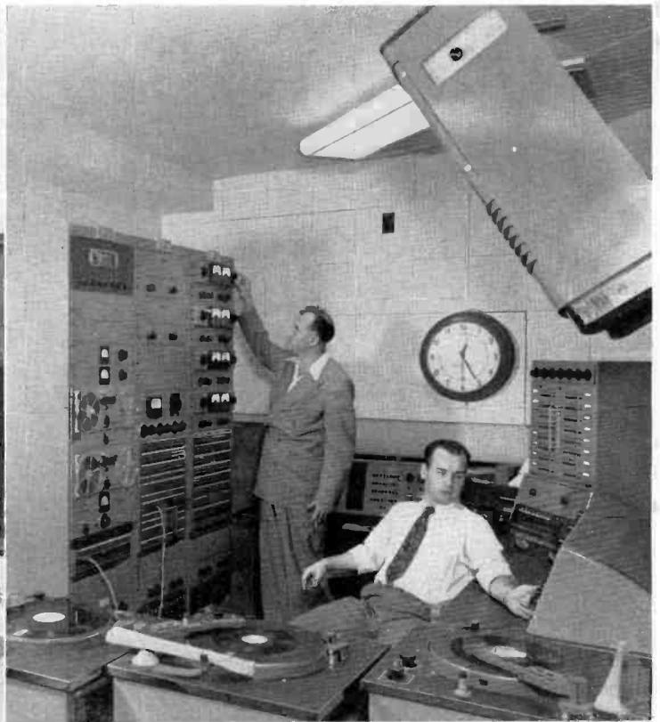
FIG. 15. Located behind the control console, are the racks of audio equipment. Mr. John M. Sherman points to the meters used to monitor regional and network AM lines.
