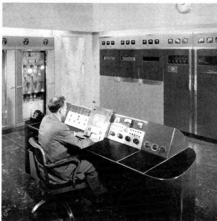
FIG. 13. View from the transmitter control room through the lobby window to the reception desk just inside the street entrance. Monitoring and test equipment units are mounted in racks at the left. Another view of the transmitter control room is shown in Fig. 6.
