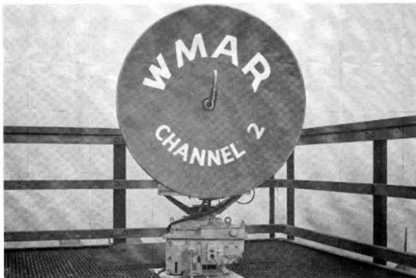
FIG. 14. Standard microwave relay dish, mounted on a Navy surplus radar base, permits remote control of horizontal and vertical positions.
