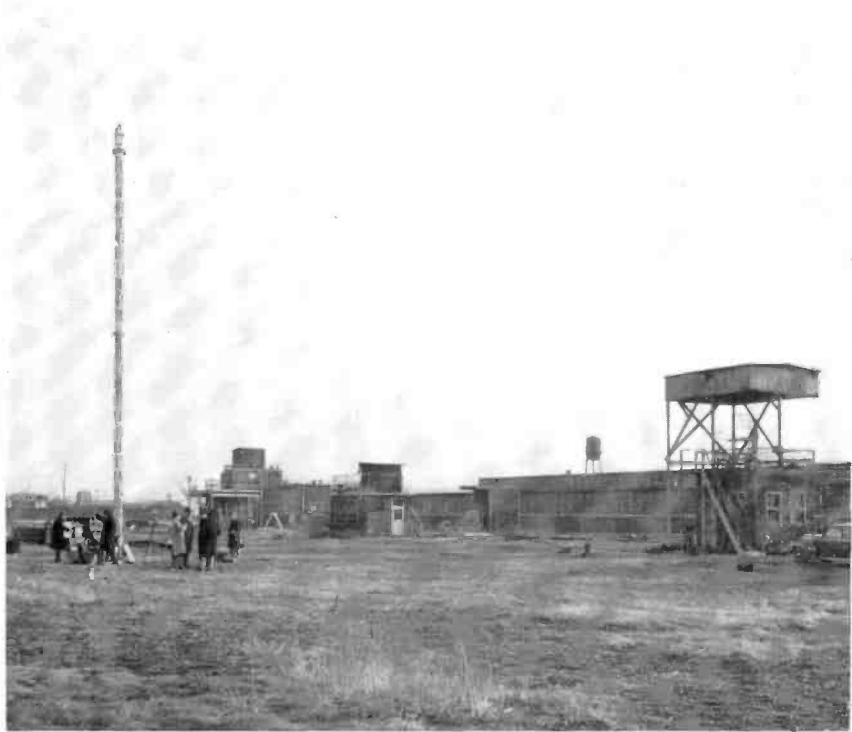
FIG. 7 (above, left). STOVEPIPE INSIDE doesn't look like a stovepipe, as this view shows. The 10-inch diameter pipe has 88 slots in its 40-foot length. Slots, which are the radiating elements, are an electrical half-wave long, are fed from inside, as can be partially seen in this end view of the top of the radiator.
