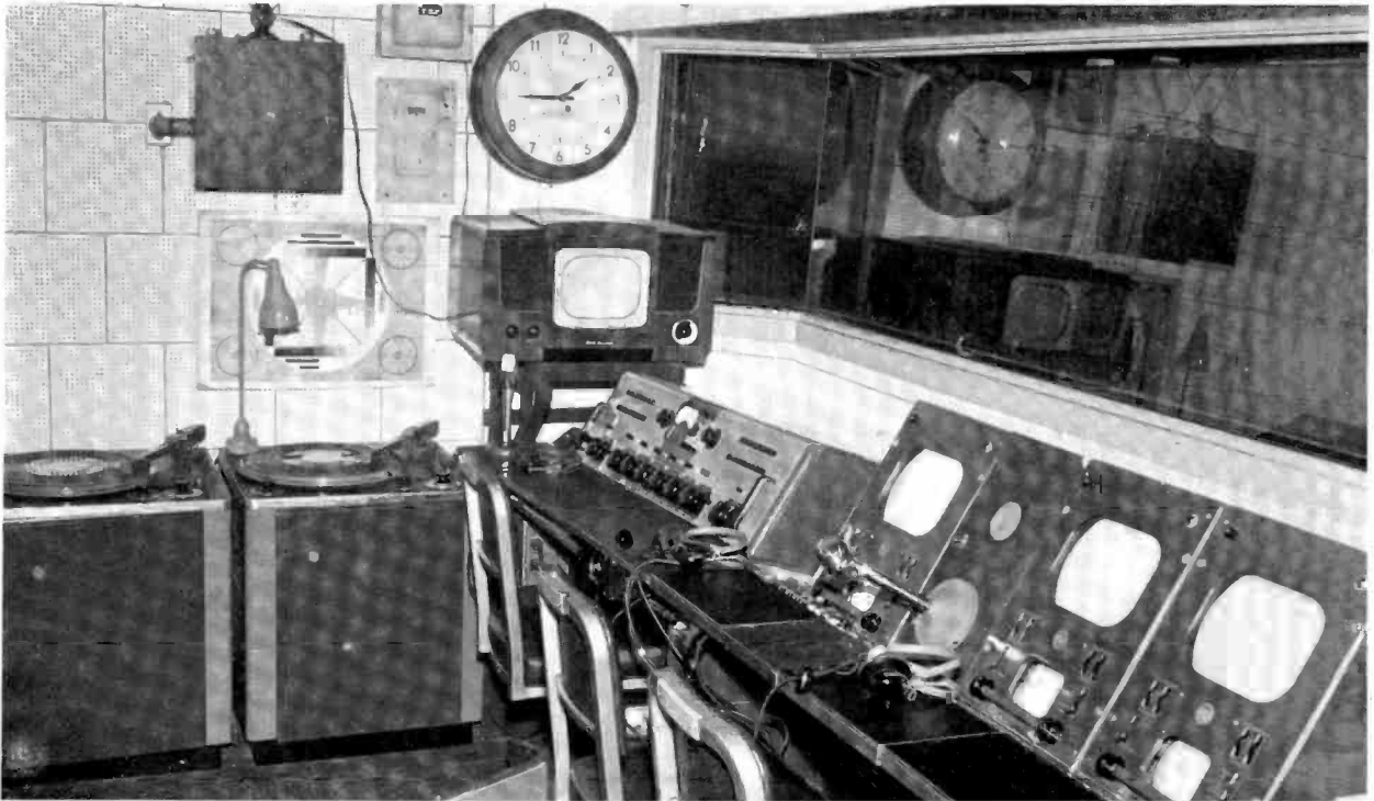
FIG. 6. Studio control room contains two camera controls, a TV switching unit, RCA Type TS-10A, Audio Console, Type 76-B4, and two 70-D Transcription Turntables. TV receiver is used as "Off-Air" monitor.
