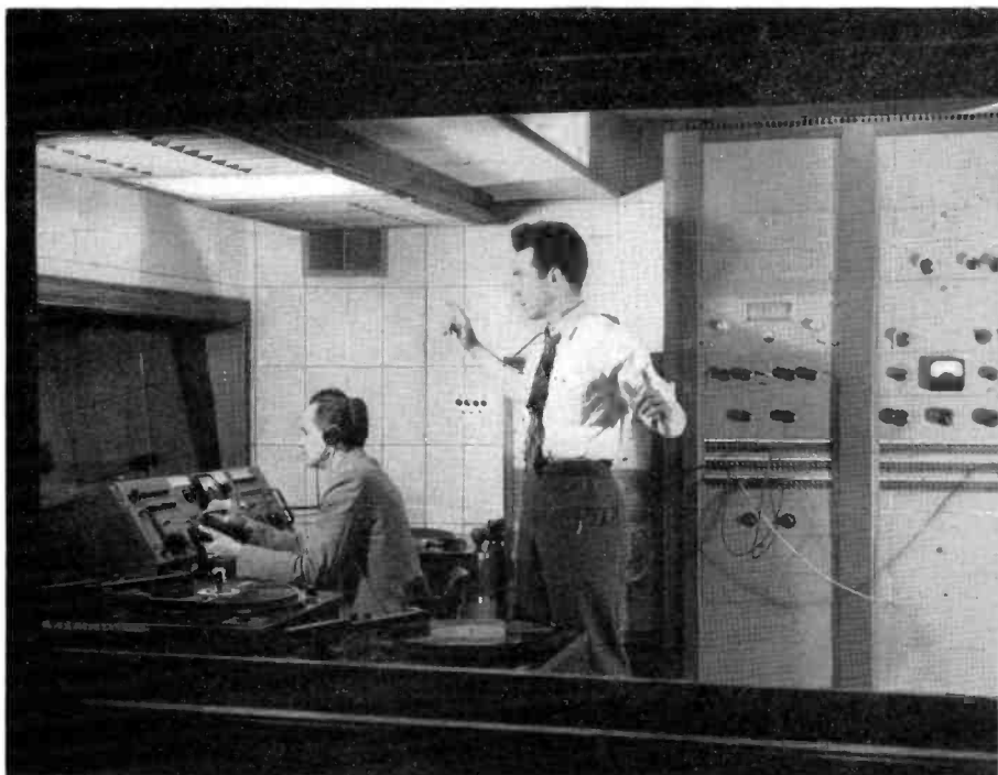
FIG. 6. Photo of studio control room taken from Studio B shows Program Director Frank Brink giving familiar cue to Studio A. Announcer-control Engineer Merrill Mael is at the controls of the RCA 76-B4 Consolette.
