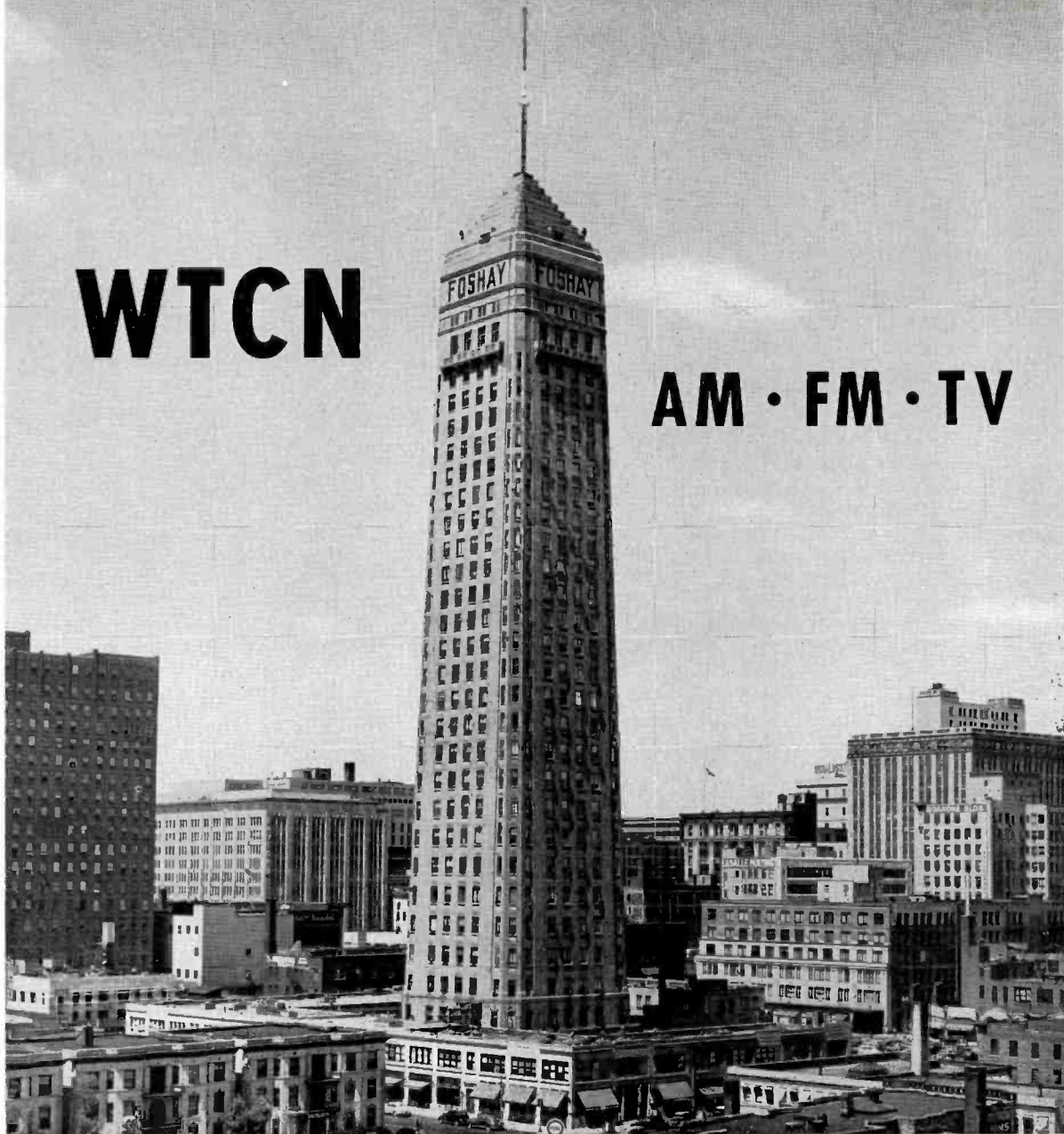
FIG. 1. The Foshay Tower Building, which is the tallest building in the Minneapolis-St. Paul area, houses the WTCN transmitters for FM and TV. The top of the tower is an ideal location for the stacked transmitting antennas and for the microwave relay receivers.
