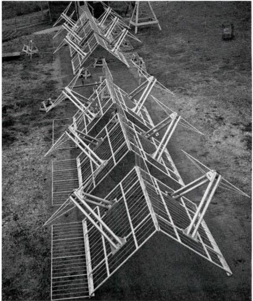
FIG. 7. Photo shows units of KRON-TV Supergain Antenna before air-shipment to the San Francisco Station. These radiator elements for KRON-TV are designed for stacking on two adjacent sides of four-sided tower as shown in Fig. 15.
