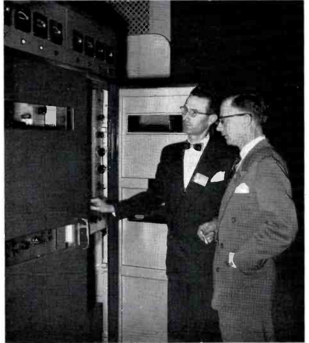
E. C. Frase, Jr. (right), Chief Engineer of WMC, WMCF and WMCT, Memphis, Tennessee, discusses features of 2-kw TV Transmitter with P. G. Walters, RCA Sales Representative, Atlanta.
