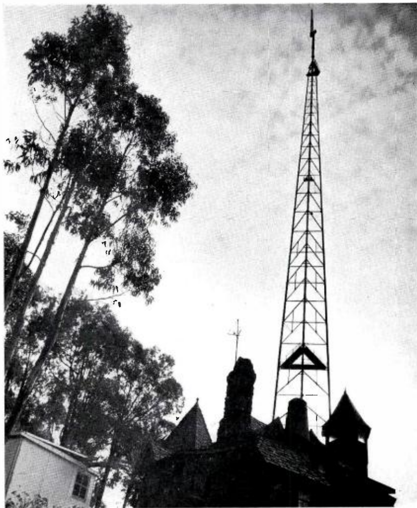
FIG. 1 (at left). The 450-foot TV-FM antenna and tower is the only outward sign of the transition of the fabulous Suto Mansion into the ultra-modern home of KGO-TV.
