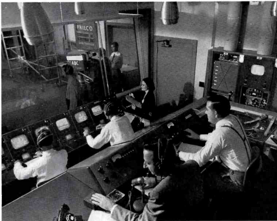
FIG. 3. Looking out on studio A. KGO-TV's control room A is built on two levels—the lower for video and the upper for audio—giving all personnel an unobstructed view of the studio.
