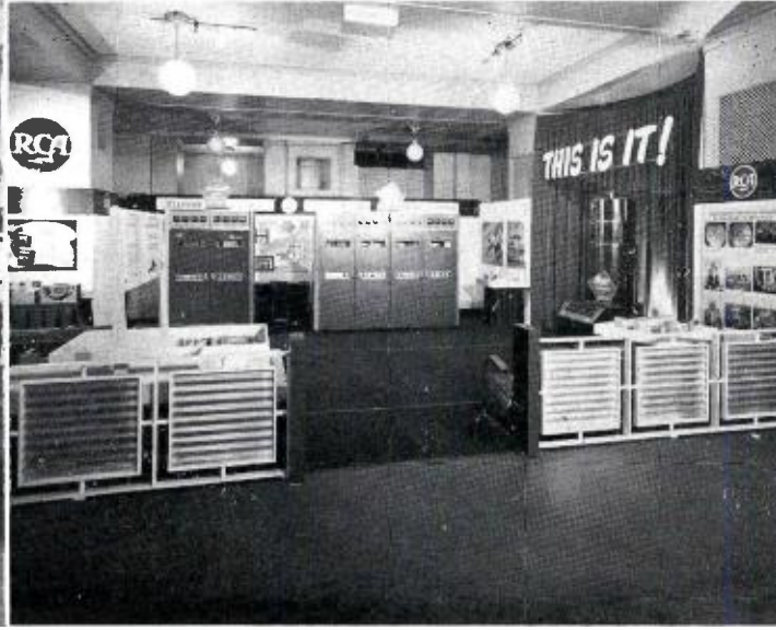
THE RIGHT WING of the booth was devoted exclusively to "TV". Displays included the new 2-kw TV Transmitter, new 20-kw TV Amplifier, plus 500-watt Transmitter and several complete TV station model layouts.
