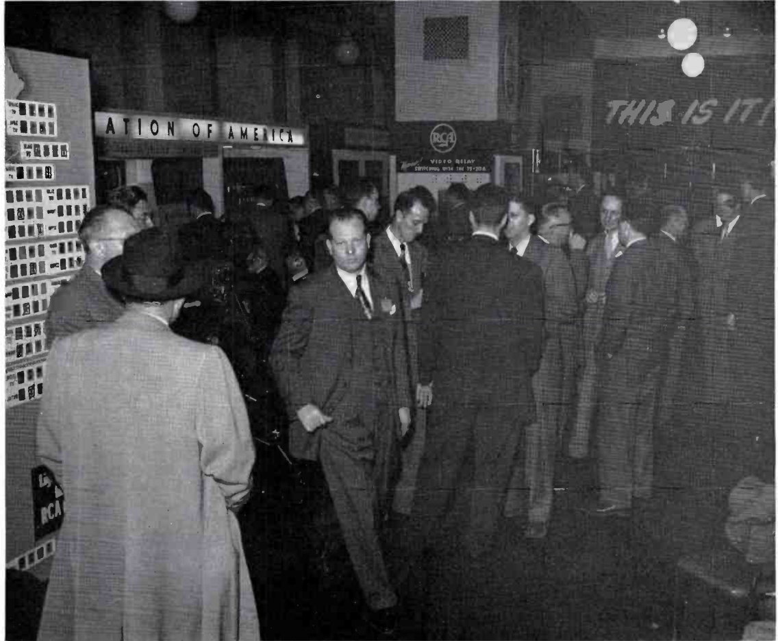
A view of part of the RCA space looking down the main aisle. Just visible at far end is the "This is it" display of the 20-kw TV Amplifier.
