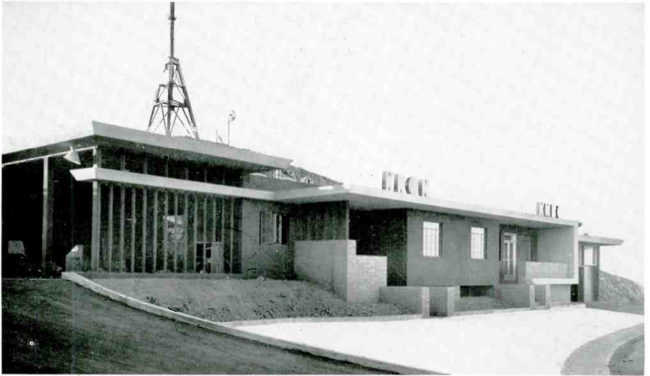
FIG. 16. View of the KRON-KNBC all-concrete building which is situated atop San Bruno mountain.
