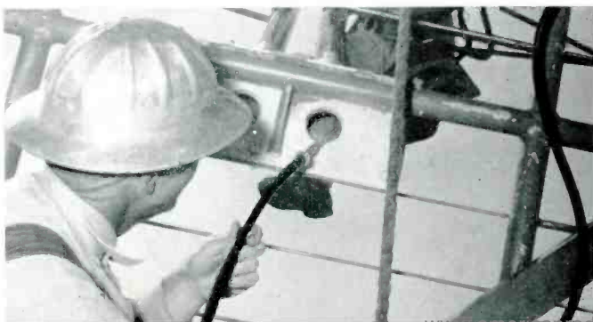
FIG. 14 RG 34/u cables were supplied with threaded brass sleeves attached to the shield braid for connection to the end of the dipole feed section. The center conductor was soldered to a fitting which connects to a strip of metal for feeding the other half of the dipole. The workman has attached the cable to a special "fishing line" so that it can be pulled up to connect to the dipole.
