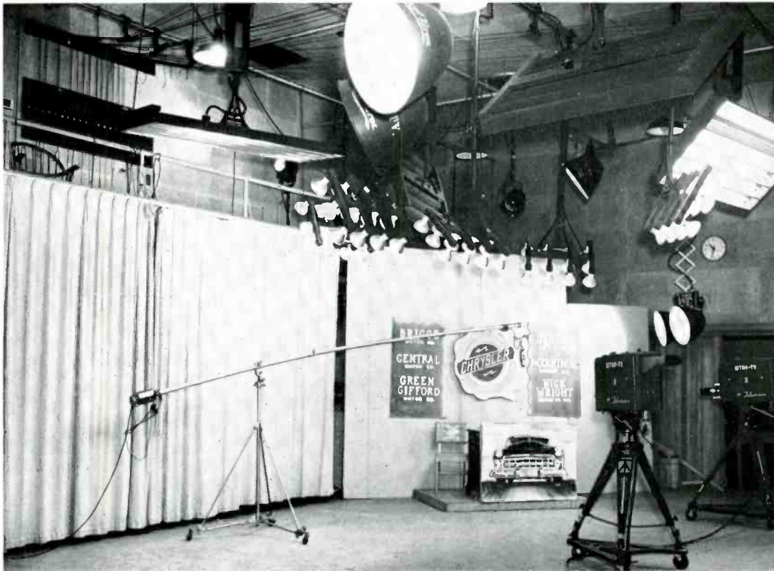
FIG. 8. This shows another corner of WTAR-TV's studio with the steel catwalk in the background. From this point the lighting man can switch the lights on or off and rotate same vertically or horizontally.
