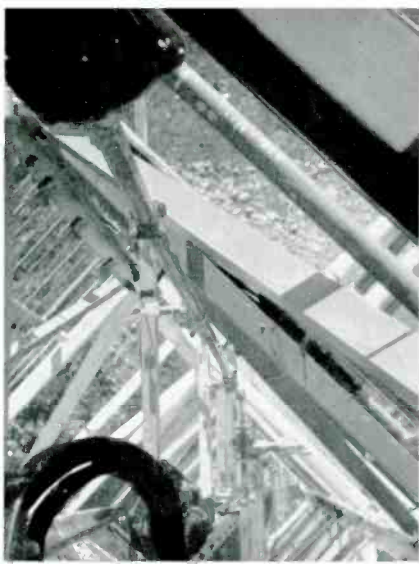
FIG. 9. Top view of the junction boxes and transformer assemblies for the TF-DA antenna. Each junction box has six RG 34 U cables of equal length which terminate at the dipoles. Coaxial transformer assemblies are made up of sections having different size inner conductors.
