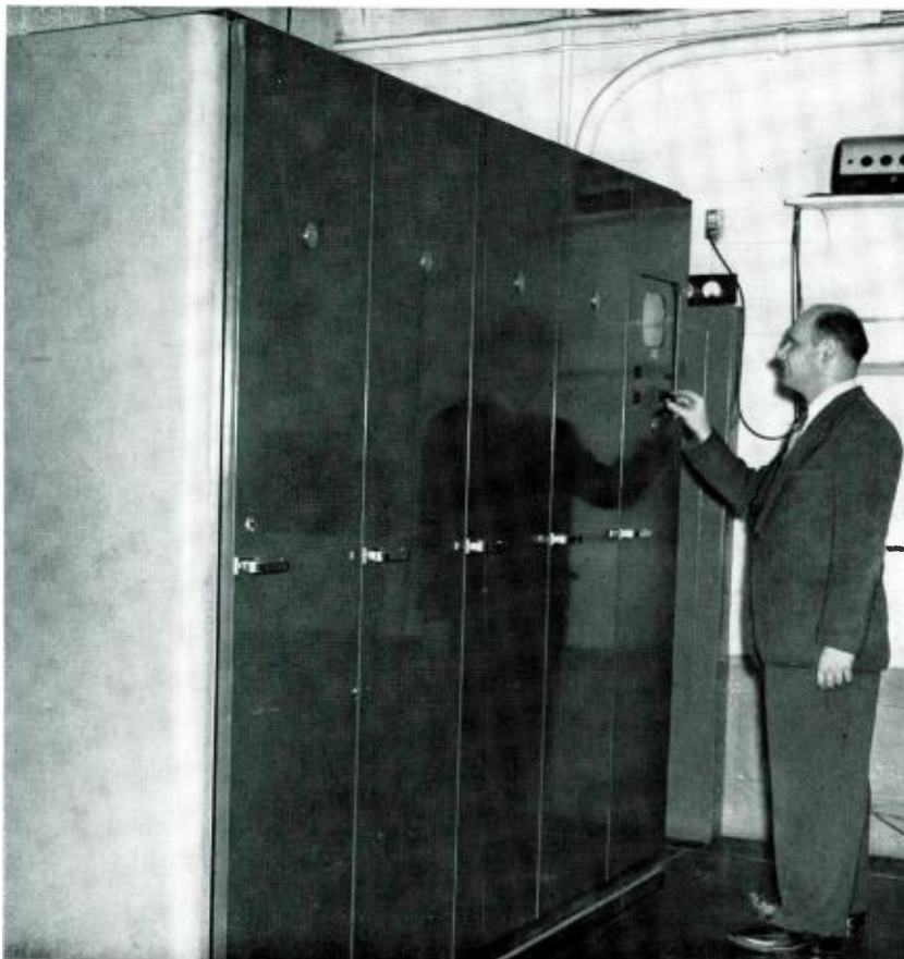
FIG. 5 (below). Operator adjusting Rack-Mounted Television Receiver.
