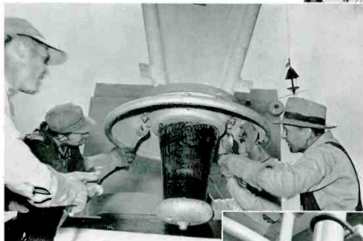
FIG. 3. The ten-inch insulator cone at base will support the entire 90 tons of KNBC's new vertical radiator tower. The tower shown in the background is part of the old antenna and was kept intact for use during construction of the new radiator. It is now available for future emergency use.
