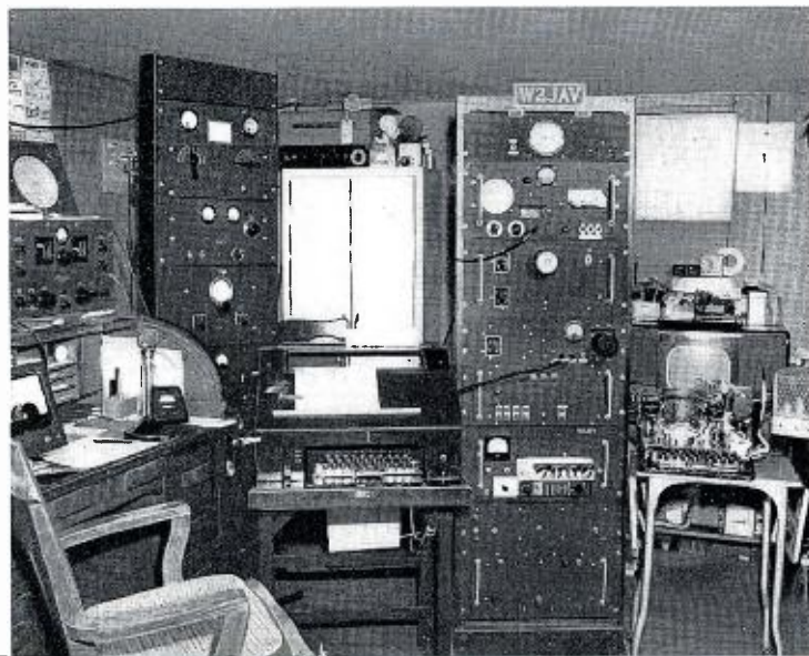
The rack in the center of the W2JAV operating room contains the original teletype gear which has been superseded by the very small unit partially visible at the extreme right. To the left of this is a teletype Model 14 tape printer, and on the left side of the rack is a Model 12 roll printer. The rack in the background is Phil's low-frequency transmitter.
