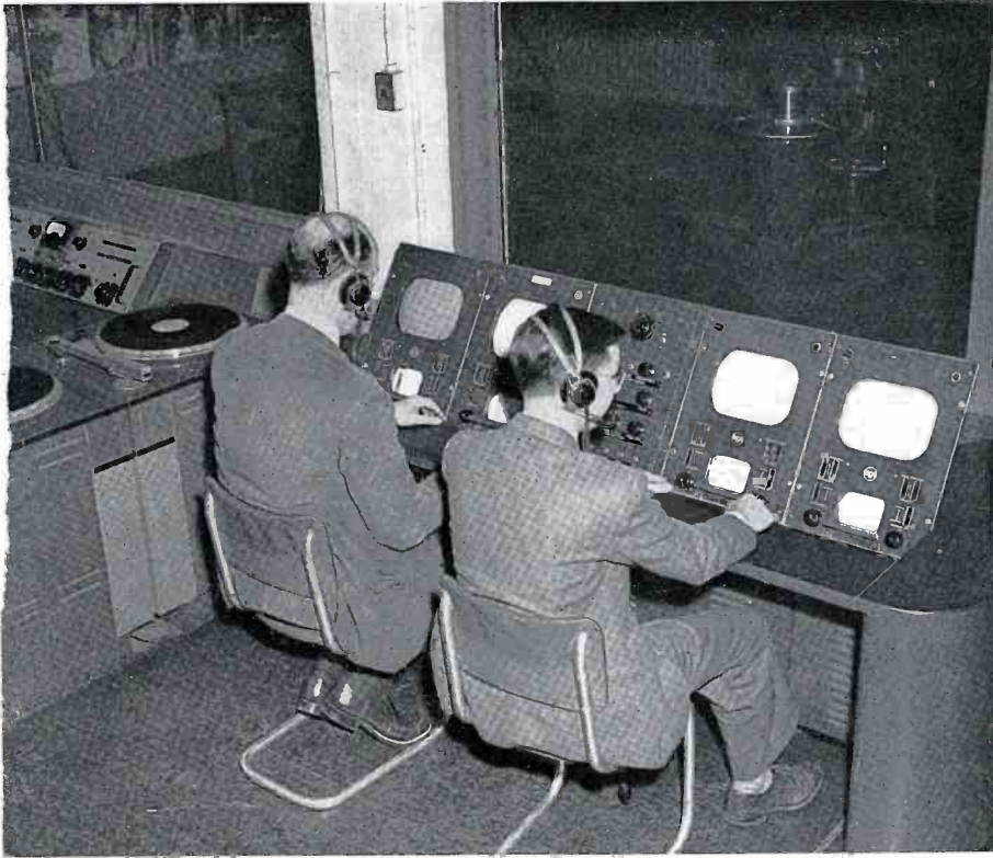
FIG. 3 (at left). Video Console containing Camera Controls, “Studio B” Switching, and Master Switching Preview Monitor.
