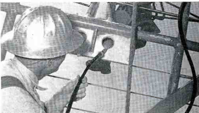
FIG. 14 RG 34/u cables were supplied with threaded brass sleeves attached to the shield braid for connection to the end of the dipole feed section. The center conductor was soldered to a fitting which connects to a strip of metal for feeding the other half of the dipole. The workman has attached the cable to a special "fishing line" so that it can be pulled up to connect to the dipole.
