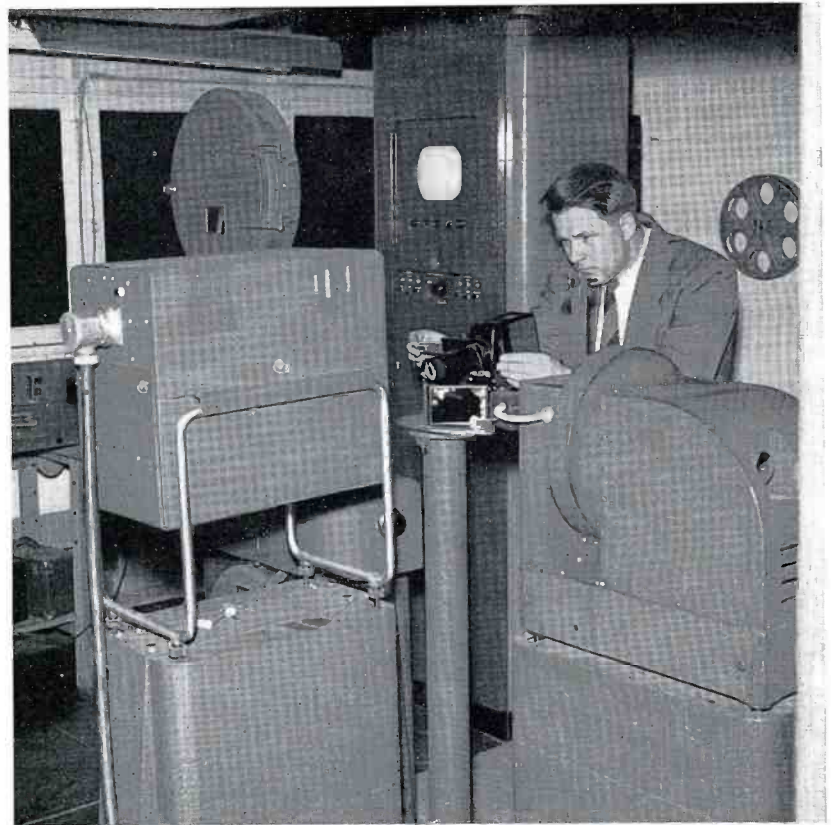
FIG. 3 (at left). Video Console containing Camera Controls, “Studio B” Switching, and Master Switching Preview Monitor.
