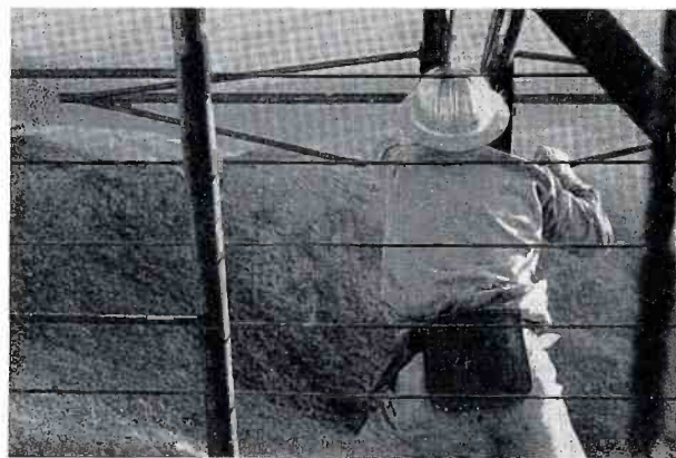
FIG. 13(A). All electrical connections to the antenna were made by erectors under the chief engineer's supervision.
