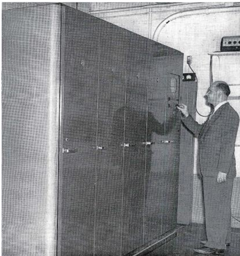
FIG. 5 (below). Operator adjusting Rack-Mounted Television Receiver.
