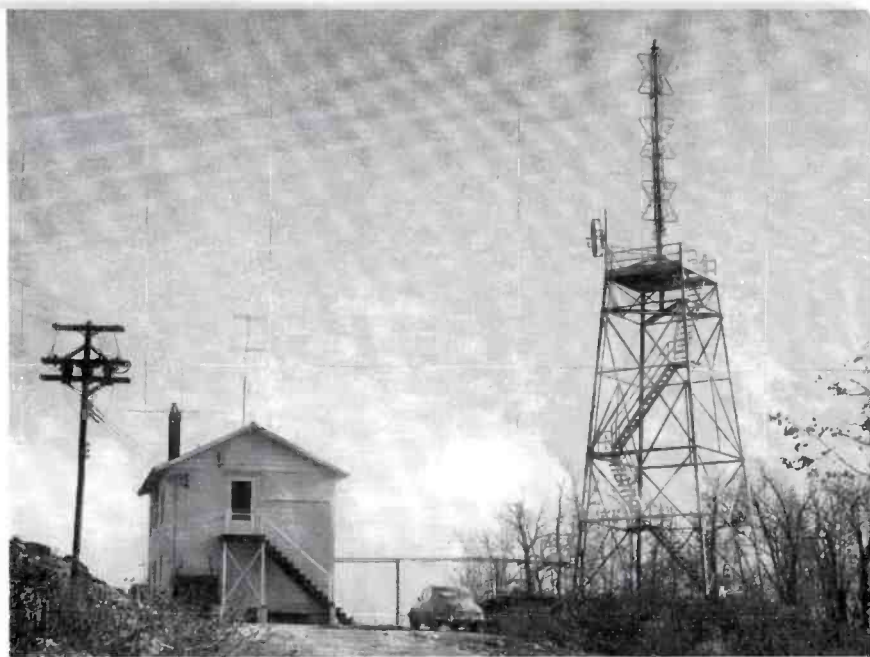
FIG. 3. Transmitter house, FM antenna and relay facilities are located about fifteen miles southeast of York.
