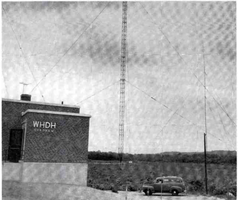
Effective 1/4 wave vertical of W1TOP is shown in above photo behind WHDH station wagon.
