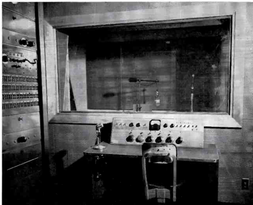
FIG. 8. In the photo of Studio D (below), one looks directly into the announce booth, containing another unit for disc-jockey operation. The Sub-Control Console shown here duplicates the Studio B control built into Master Control, with the exception that "B" microphone is built in. Since the announcer controls his own turntables, only one turntable control is needed here.
