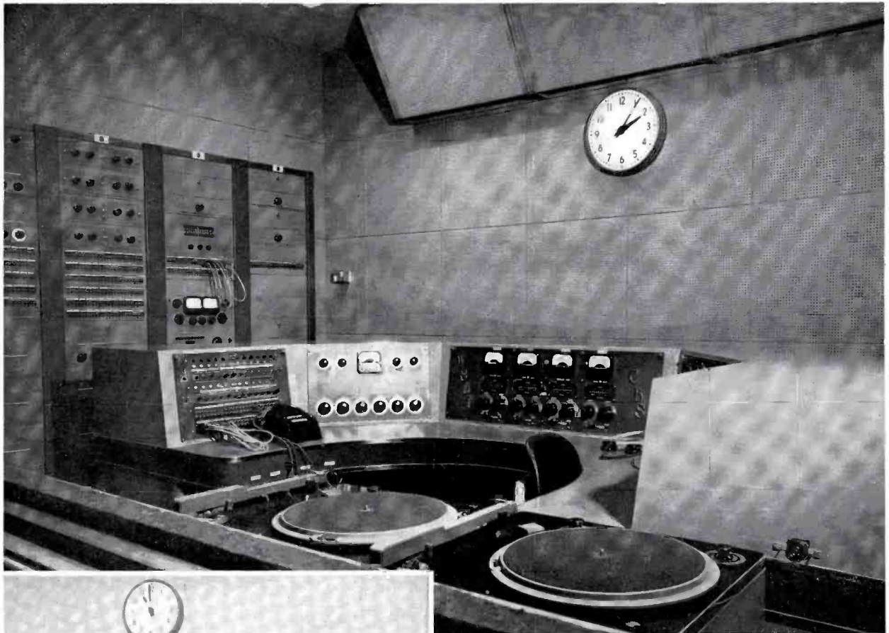
FIG. 3. The Master Control Console is an RCA custom unit, designed for great versatility. The left-hand panel handles the telephone ring-down circuit for 24 remote program lines which can be patched into jack panel. Four lines go to each studio, and four order wires to remote locations. The buttons are for feeding cue to any of the remote lines.
