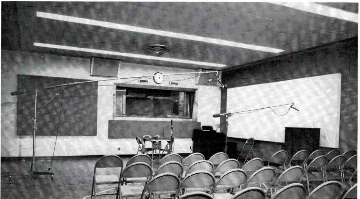
FIG. 6. This is a view of Studio A which seats an audience of approximately 100 persons. The station's call letters are inlaid on the floor. The LC-5A Wall Speakers are here shown mounted at the proper angle for a long throw — as is needed in this room.
