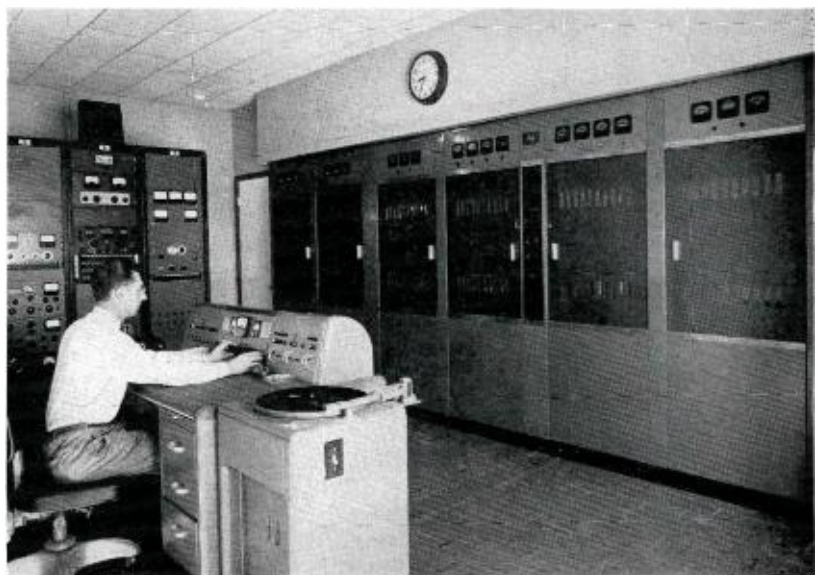
FIG. 4. View of KSOO transmitter room showing RCA BTA-10G with matching phasing cabinets to the left. Audio control racks can be seen at extreme left. Mark Boese, KSOO engineer, is seated at the controls.
