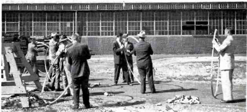
FIG. 2. Prefabricated lengths of Styrolflex Feed Line being prepared for antenna assembly.
