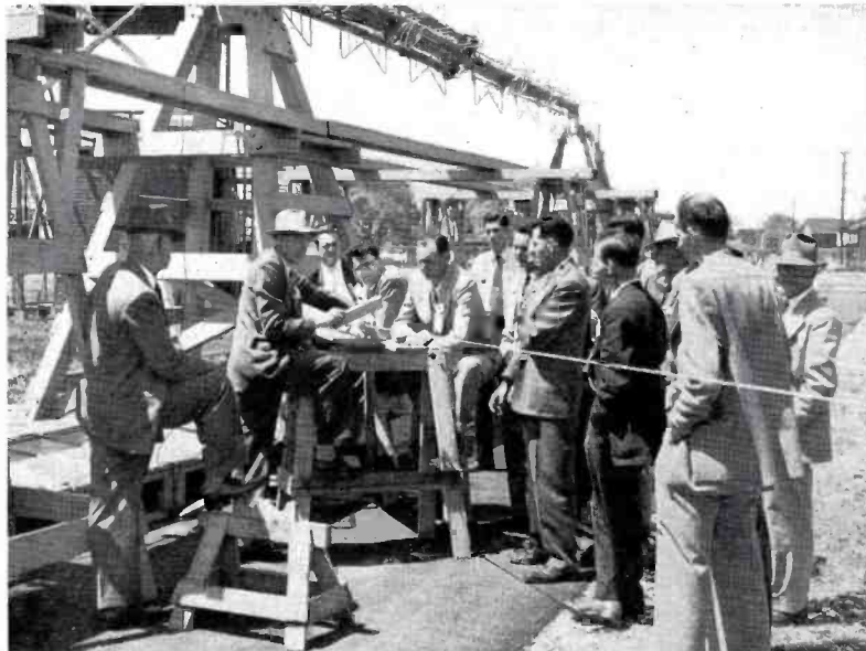
FIG. 7. W. F. Hanson, RCA, demonstrates the effect of standing waves on transmission line.
