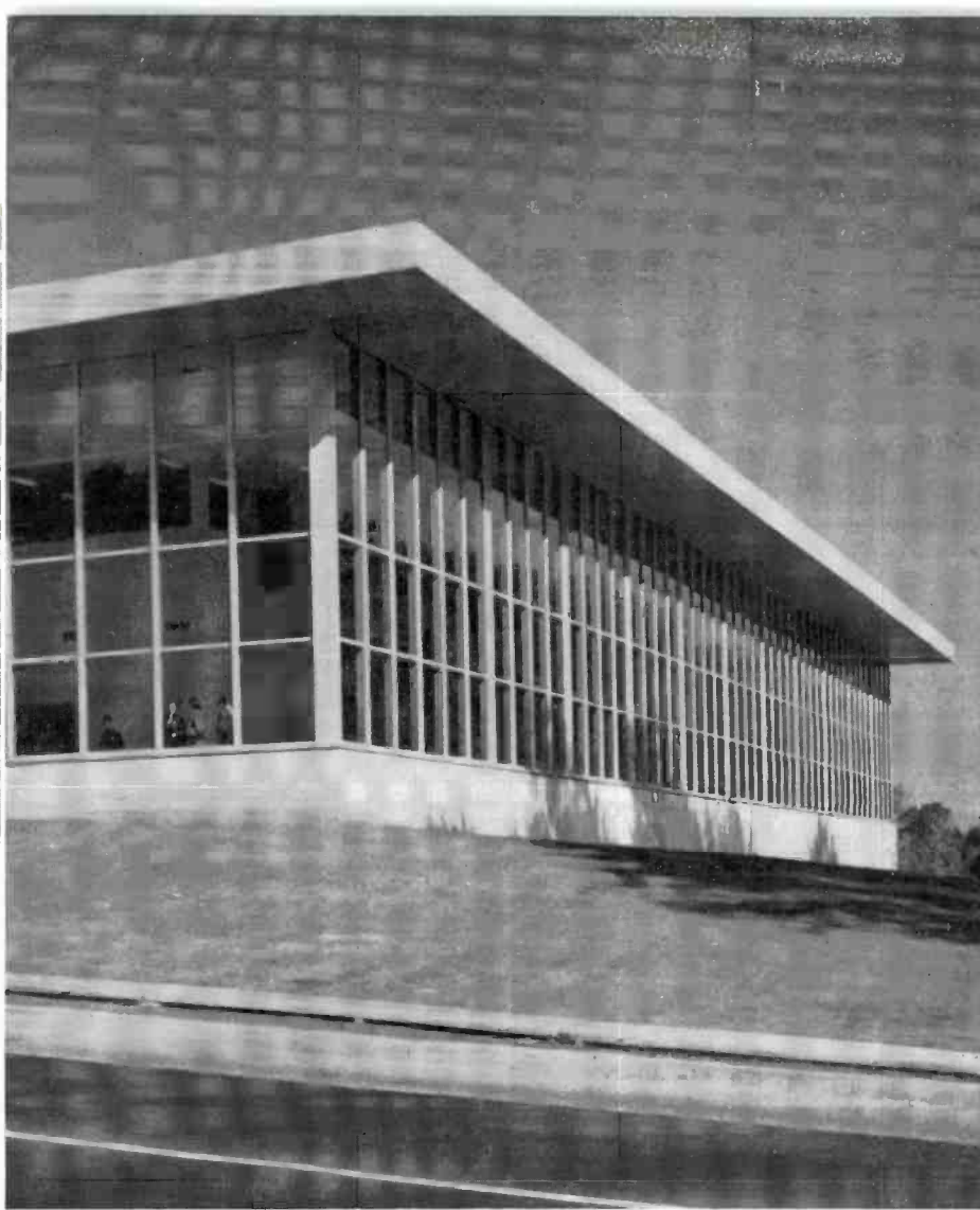
FIG. 1 (left). WCAU's new Radio and Television Center is an ultra-modern building 201 feet wide, 220 feet deep and the equivalent of three stories in height. The building is completely air-conditioned and is windowless except for the south and east walls of the lobby which are entirely of glass.
