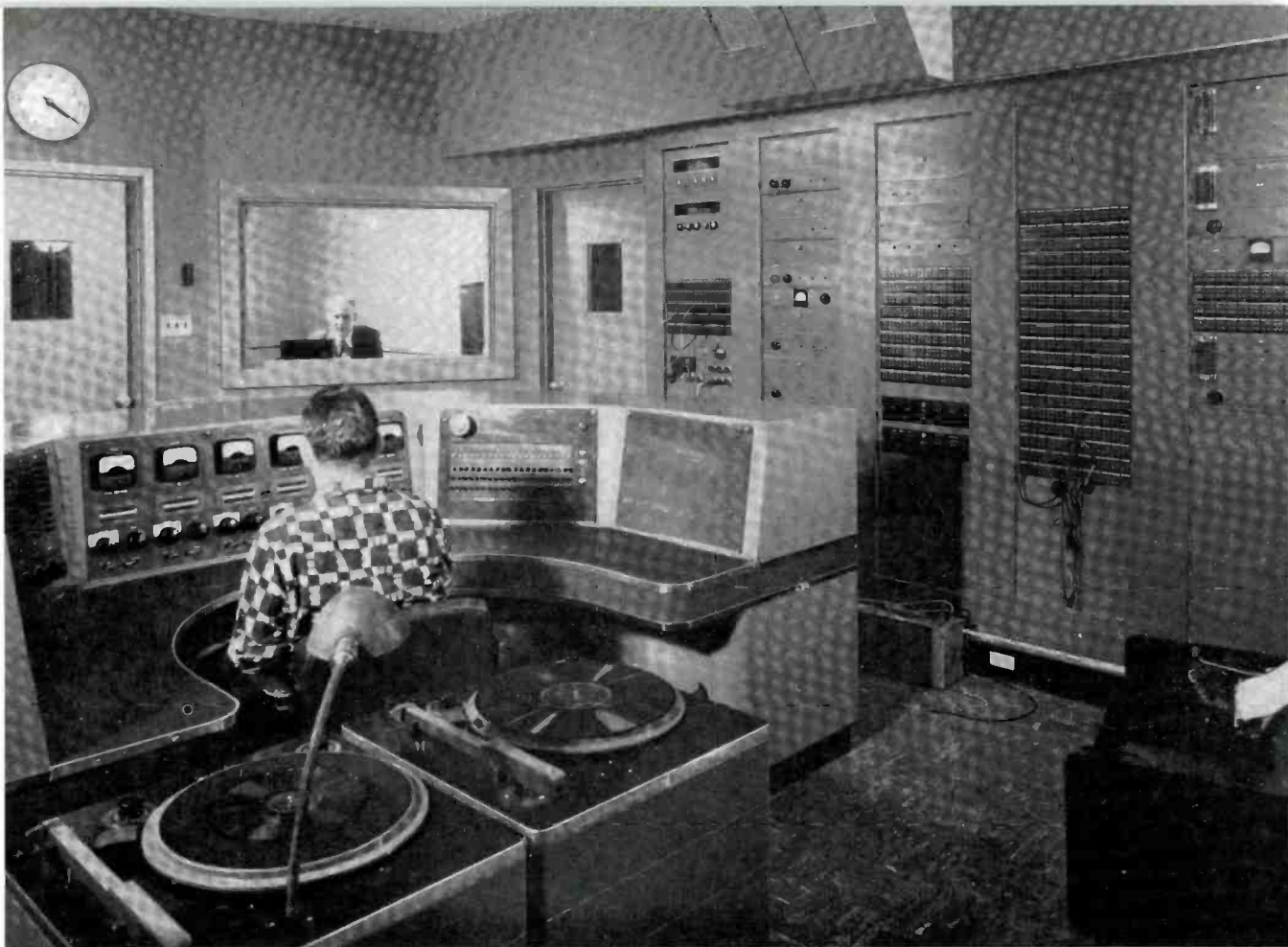
FIG. 44. Radio master control room at WCAU. Console is a deluxe RCA unit custom built for WCAU. Racks of RCA amplifiers and other units at the right form the wall between the control room and the equipment room which is located between the radio and TV master control rooms (see Fig. 46).
