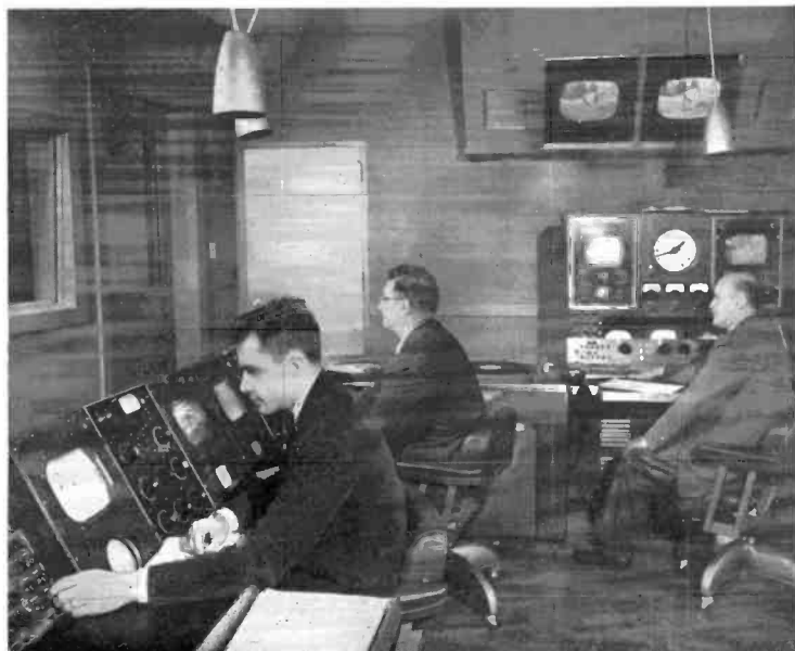
FIG. 38 (above). This is the WCAU TV Master Control Room as seen through the window from the main lobby. The film and announce camera monitoring positions are at the long console on the far side of the room. The master control switching console, especially built by RCA to WCAU's specifications is at the extreme right. The door at the left rear leads to the projection room, part of which can be seen through the window at the right of the door. The window further right looks into the announce booth, and through a second window into the part of the projection room where the announce cameras are located. The floor arrangement of this section of building is shown in Fig. 46.
