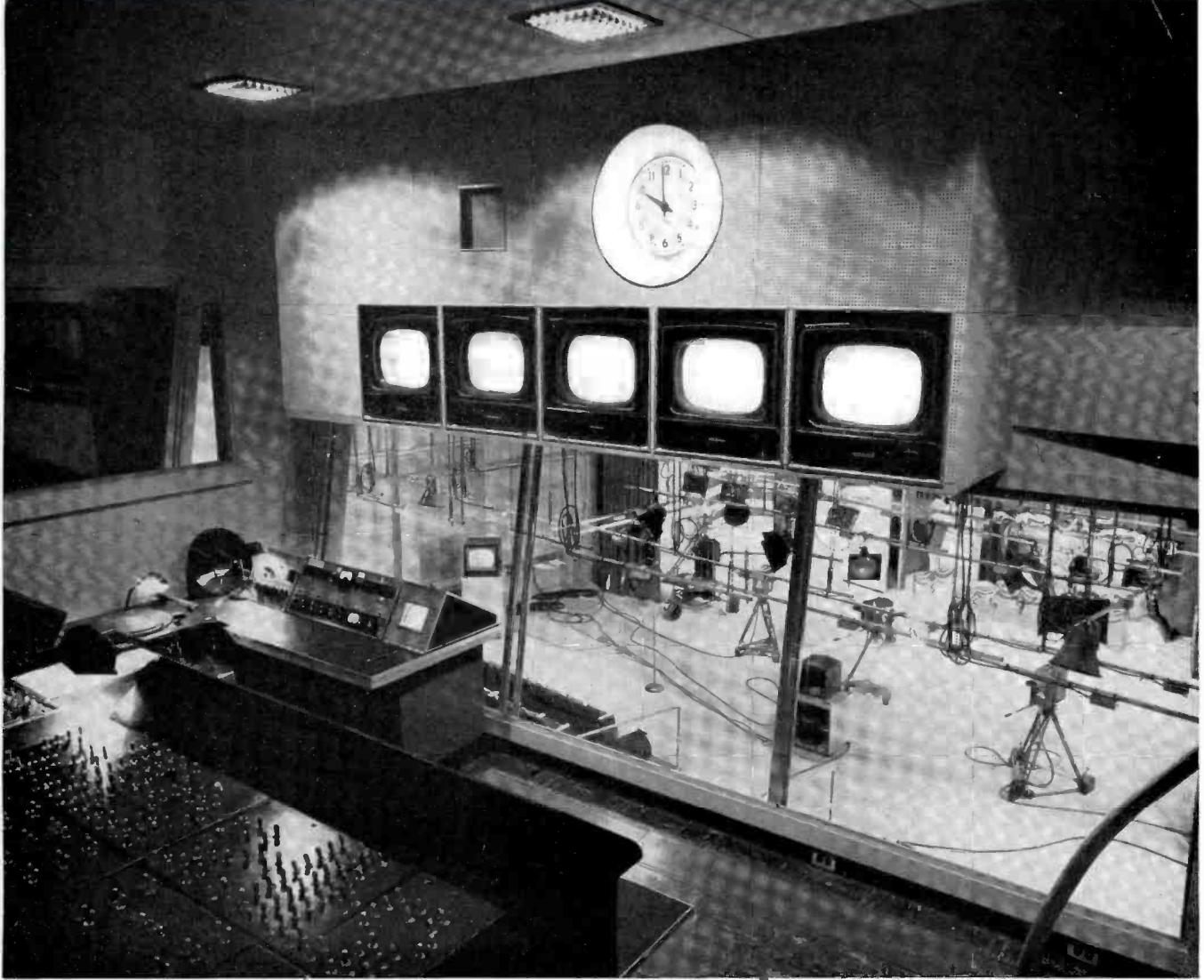
FIG. 29 (above). The control rooms of all three TV studios are practically identical. A 6-foot high Solex glass window the full width of the control room, plus the elevated position, gives unequalled visibility of the whole studio. Another unusual feature is the fact that only the audio operator is on the lower level. He sits at a console which consists of an RCA BC-2B Consolette, an RCA OP-7 Amplifier (for extra mic positions) and a program monitor mounted in a streamlined desk designed by the WCAU engineering staff. The video operator, program director and lighting operator sit on the upper level where they can observe the camera, preview, and program pictures on the 17-inch monitors mounted above the window.
