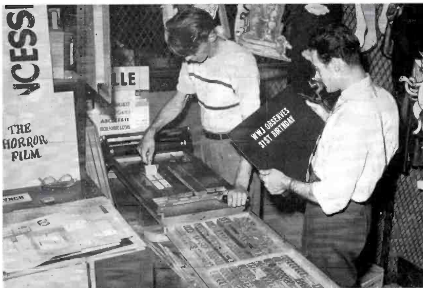
FIG. 19. A poster press similar to the type used by department stores is a graphic arts adjunct at Station WWJ-TV. As many as twelve "headlines" for a news show can be set up in an hour.
