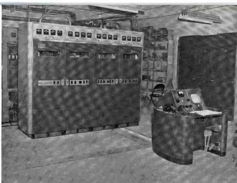
FIG. 6. Shown here is the RCA TT-2AL interim transmitter and control console. Directly behind the 2-KW unit is the TT-10AL ready for the change to higher power.
