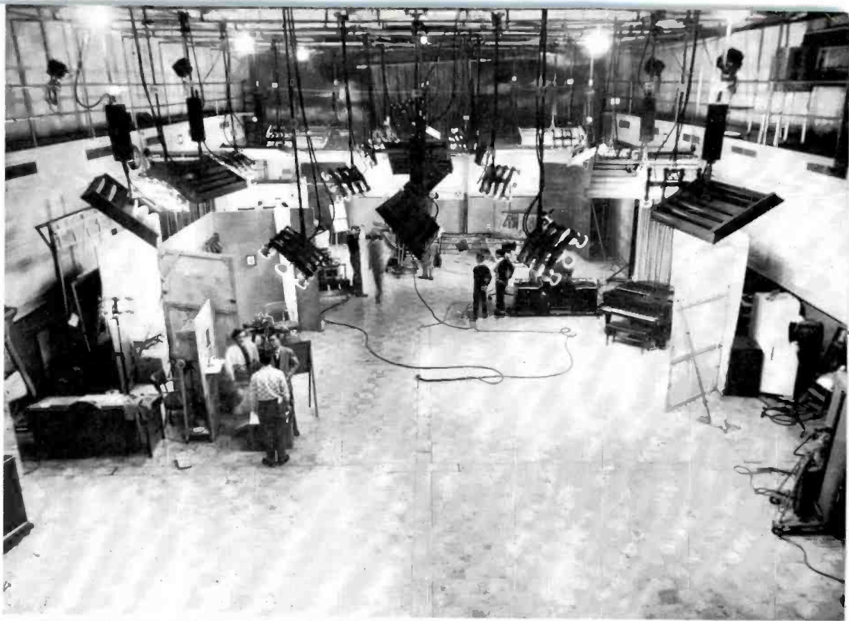
FIG. 9. This view shows the opposite end of WBAP Studio #1. All lights are suspended from a pipe framework and can be rotated by means of rope controls which are operated from a "lighting bridge" (extreme right in this picture). In normal operation a number of "sets" are arranged along the sides of the studio. Cameras, operating in the center area, move from set to set.
