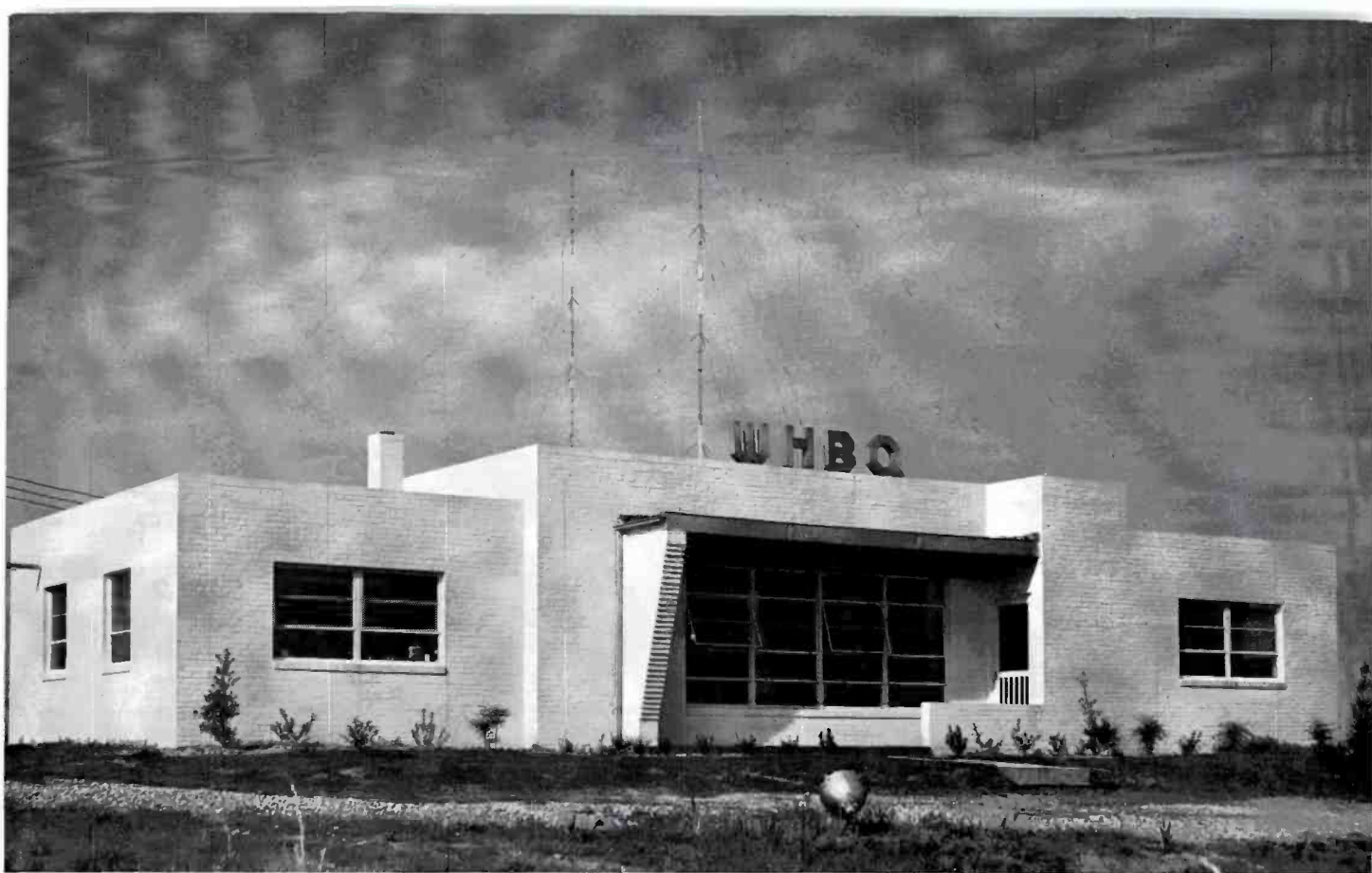
FIG. 1. The WHBQ 5000-watt transmitter building, with its solar-type front facing south. Two of the five 315-foot towers are visible in the background.
