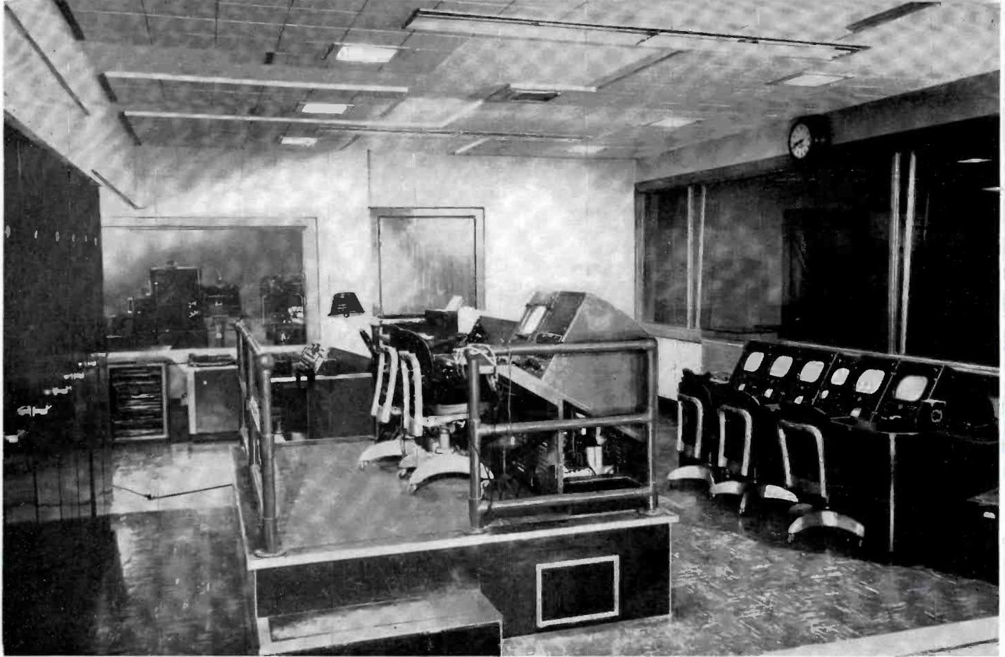
FIG. 13 (above). WBAP's television master control is combined with TV Studio #1 control as shown above. Five camera monitors (3 live, 2 film) and a preview monitor are on the lower level, next to the studio window. The program director and technical director sit on the raised platform. The TD, who does the camera switching, has a master monitor as well as the switching controls on his console. The audio operator sits at a floor-level console to the left of the program director (just behind the raised platform in this view).
