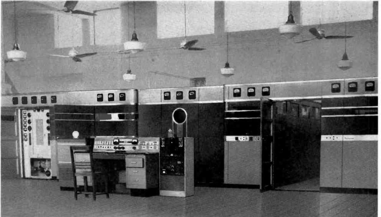
▲ View of No. 2 RCA transmitter in Radio Pakistan's Transmitter Hall. The front panels of the transmitter are designed to allow ready access to the various units of equipment. Door actuated switches connect to an interlocking system to protect personnel against exposure to dangerous voltages.
