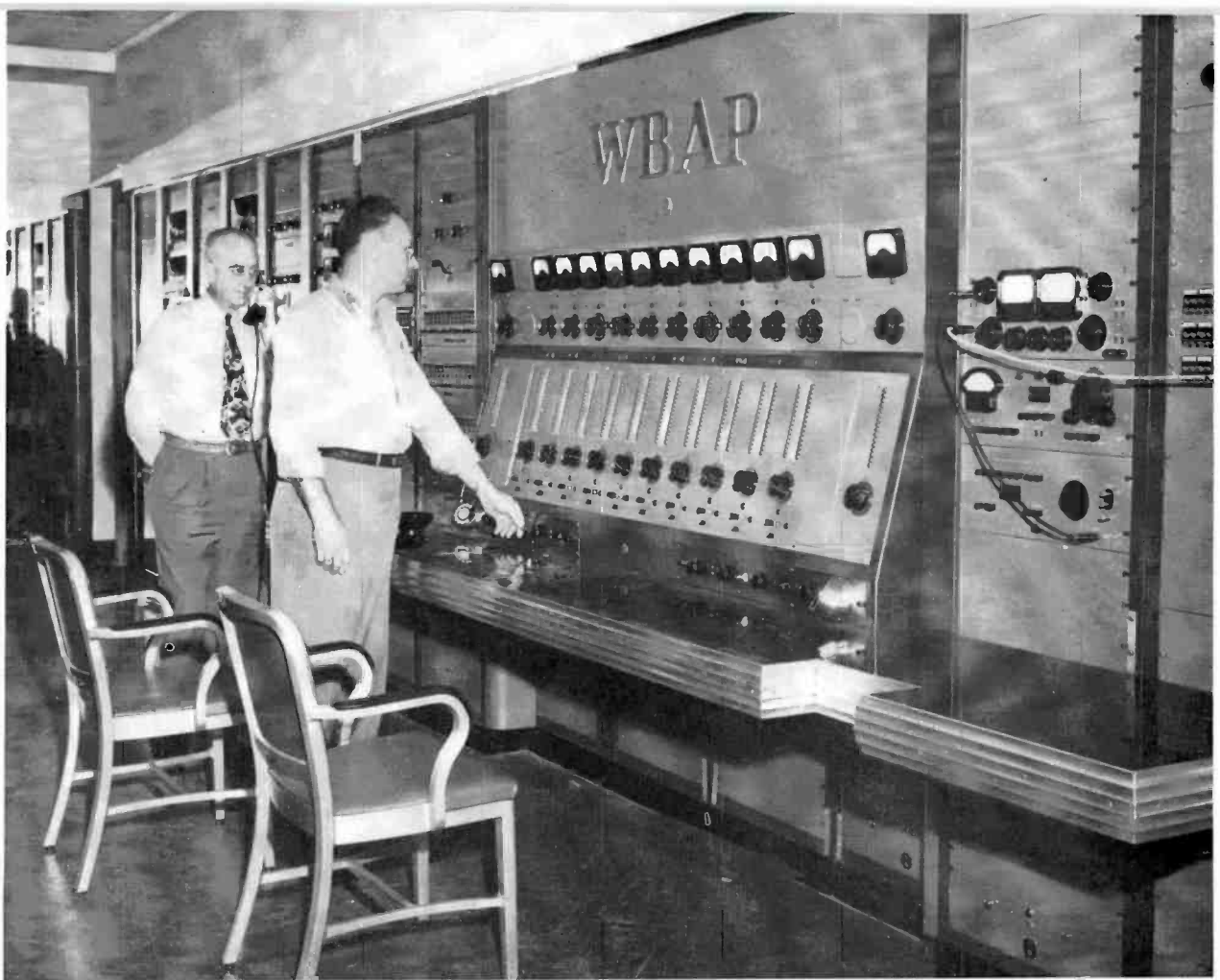
FIG. 3. This is a closeup of the main operating position of the WBAP master control position. The special four-rack-wide control section was custom-built by RCA to WBAP's specifications. It provides means of switching sixteen incoming circuits to any or several of ten outgoing circuits with complete "preset" facilities. Arrangement of controls is shown in diagram, Fig. 4, on opposite page. Operation is described in the text. Shown in this view are, at left, R. C. Stinson, Technical Director of WBAP, under whose direction this equipment was planned and installed; and, at right, Roy Bond, of the WBAP engineering staff.
