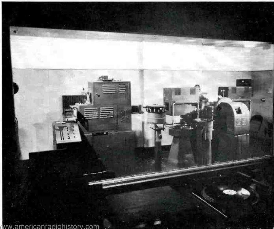
FIG. 16 (below). View looking from the control room into the film projection room. Equipment in the projection room includes two RCA TP-16D Film Projectors and two RCA TK-20A Film Cameras. The latter are mounted on revolving type pedestals so that they may be turned to face one of several projectors. In addition to the film projectors there is Grey Telop and a Selectroslide projector, with space provided for a second.
