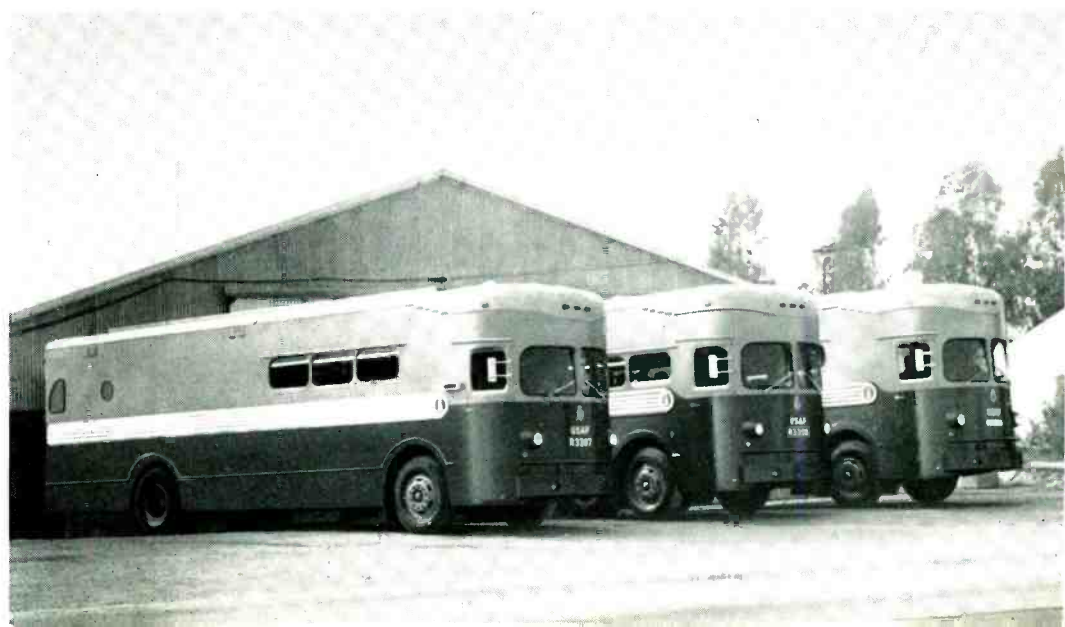
FIG. 2. Complete Television facilities are housed in three 35-foot vehicles of special design.
