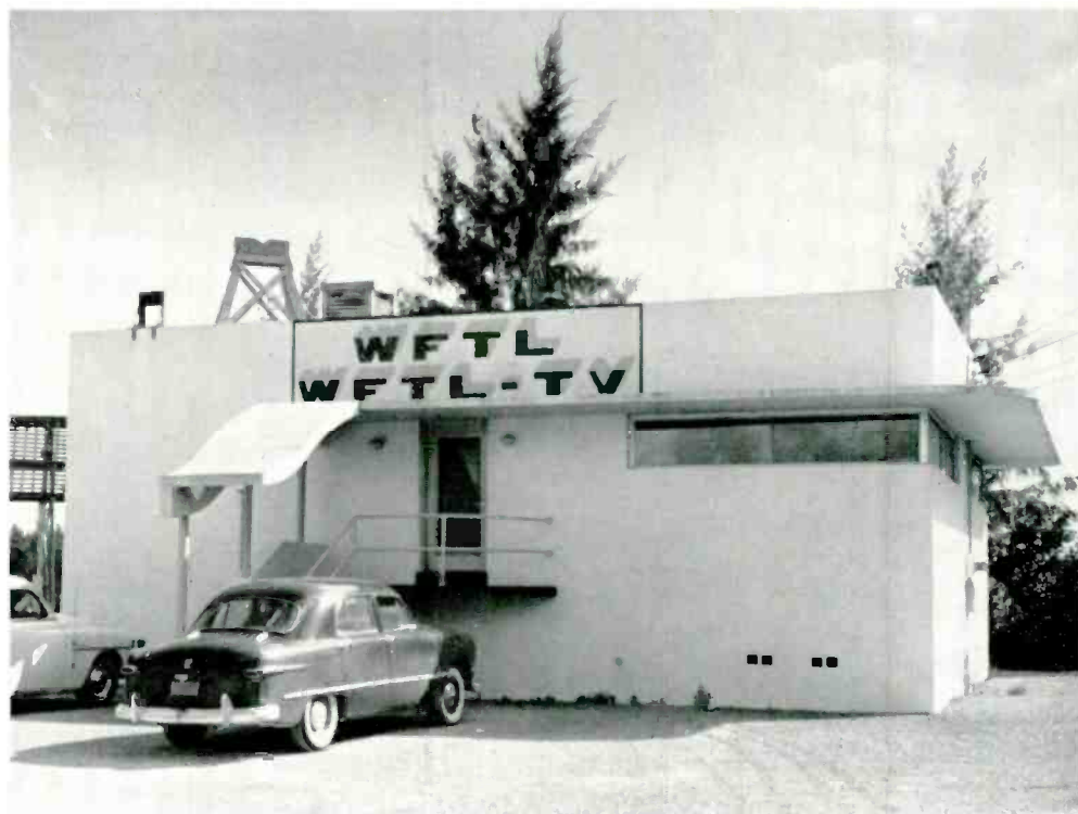
FIG. 8. Exterior view of transmitter building located at 1785 Southeast 15th Street, Fort Lauderdale.
