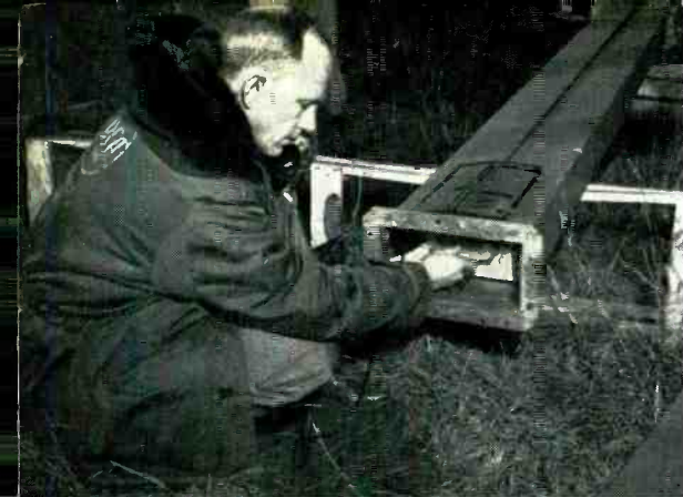
FIG. 2. F. J. McMenamin adjusts temporary shorting plate at end of a test length of waveguide (shown below, Fig. 3) for product development test.
