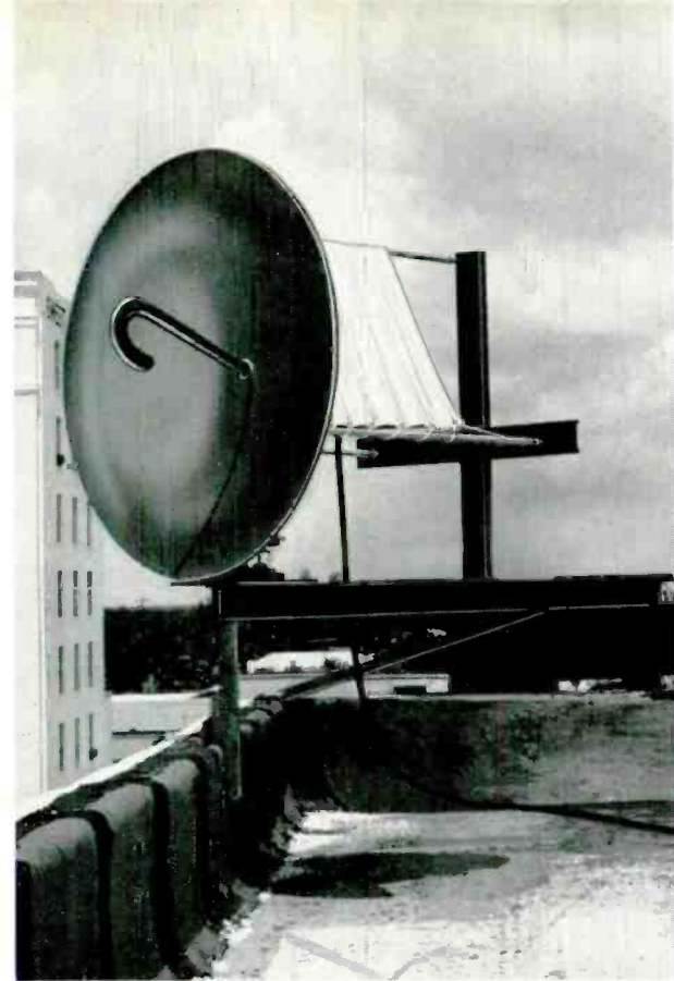
FIG. 7. Microwave transmitter "dish" atop downtown studio building delivers TV program signal to transmitter building via passive reflector and receiver dish shown in Figs. 5 and 6.
