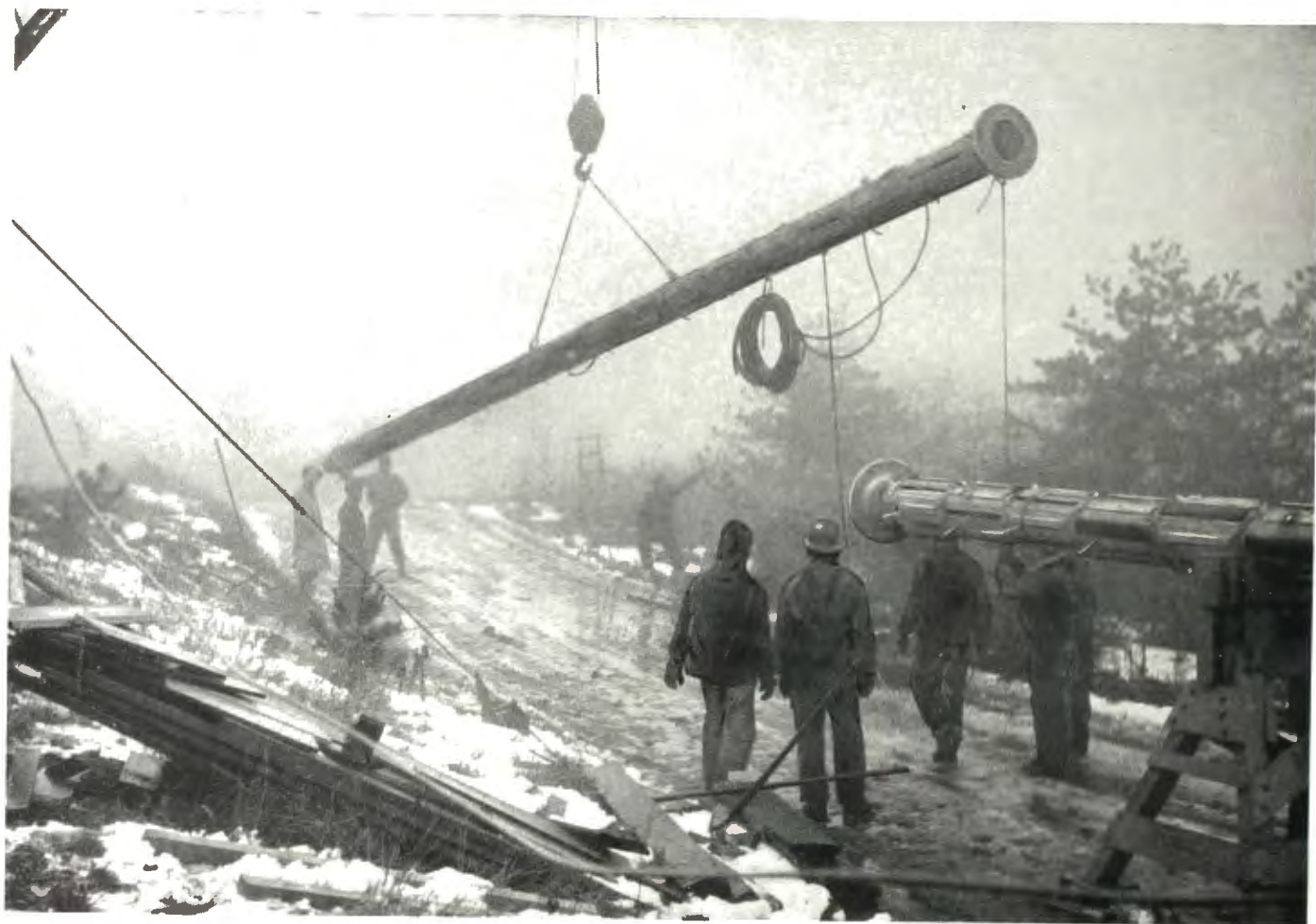
Unloading and assembling operations proceed despite cold and rainy weather. Here the top section of the antenna is being lowered into place so that the complete antenna can be assembled for a ground check at the WBRE-TV site.
