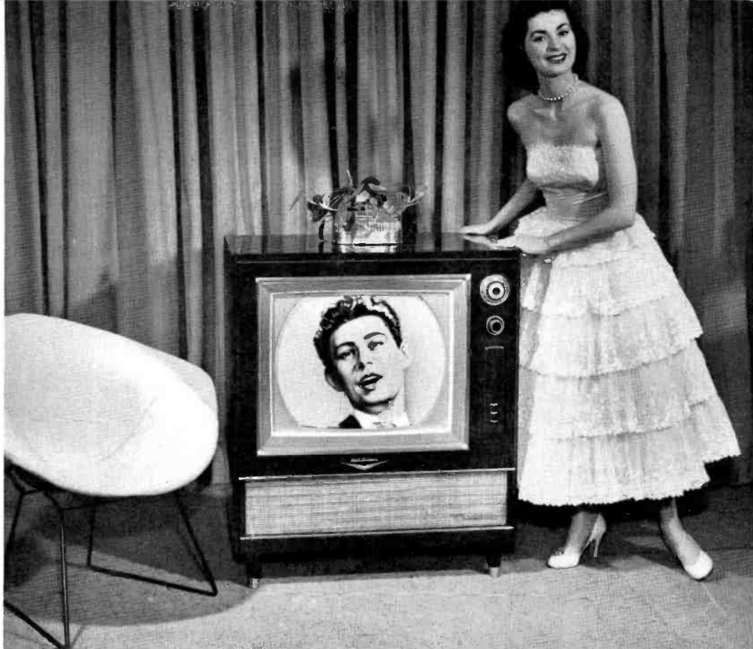
FIG. 10. This deluxe RCA Color Receiver is the "Director" (Model 21CT662), an open-face console with two 8-inch speakers. Suggested list price is $895.
