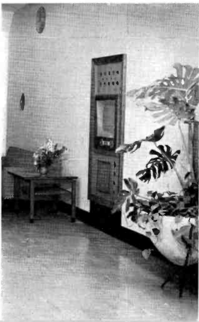
FIG. 31. House monitor located in main lobby. Receiver is mounted on runners which permit chassis to slide out for servicing.
