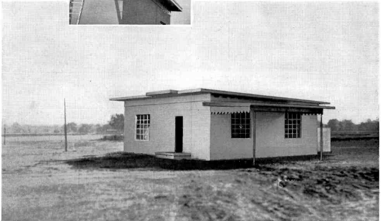
FIG. 2. The just-completed WCBI transmitter building, 32 by 32 feet, is shown in this view. Made of all concrete, and designed for future expansion on the 90 acre WCBI "Antenna Farm," the building features steel casement windows, glass wool insulation, ventilated ceiling loft, a flat-top roof and plenty of parking space. The deep well and pump house is shown at the rear of building.
