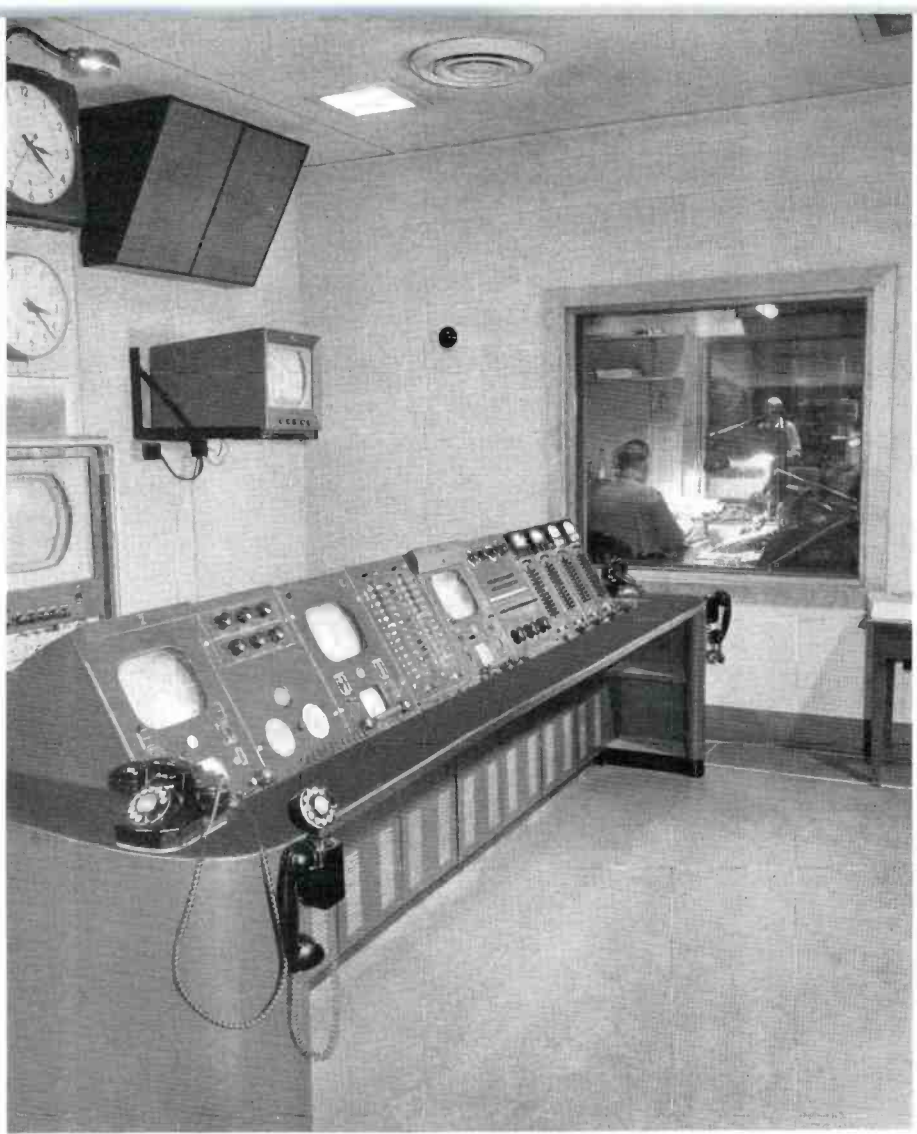
FIG. 22. Master Control facilities at this console include audio and video switching panels, master monitors and an audio ringdown and remote panel. The booth shown is the Studio "X" announce booth where any or all of the four outgoing audio channels can be overridden.
