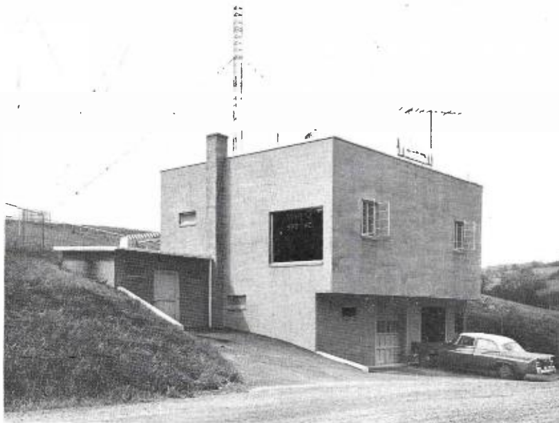
FIG. 5. The WHLM transmitter building lies in the valley between the second and third tower. It is constructed of concrete block and has more-than-adequate room for its AM and FM transmitting equipment.
