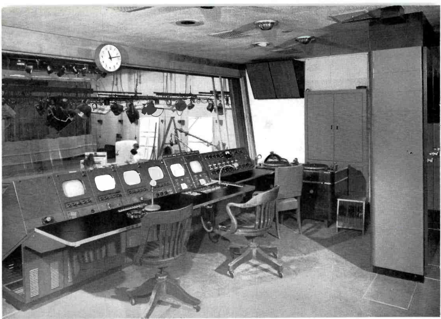
FIG. 12. Studio A control room—note equipment bays at extreme right. Control rooms B and C are similar in layout.
