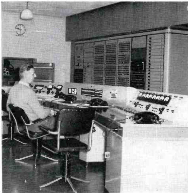
FIG. 10. Master control at Munich Studios feeds program signals to transmitters for target countries. (This unit was designed and built by RFE engineers.)
