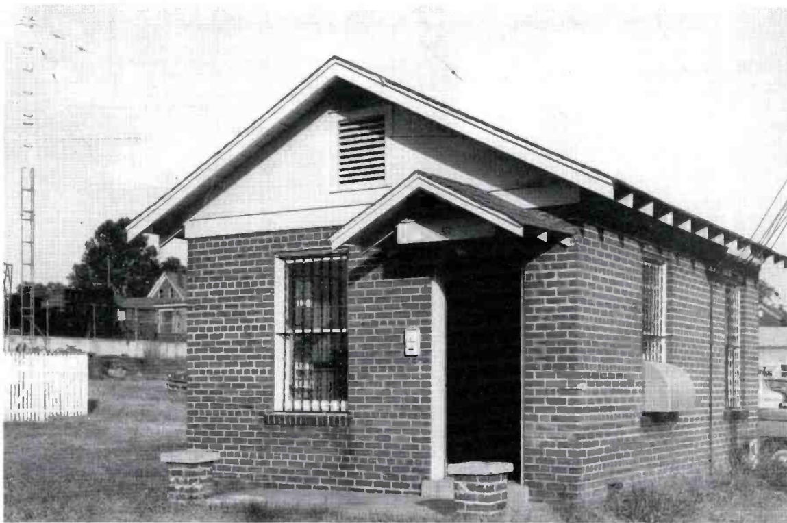
FIG. 8. Transmitter building contains a remotely controlled RCA B1A-1M AM Transmitter.
