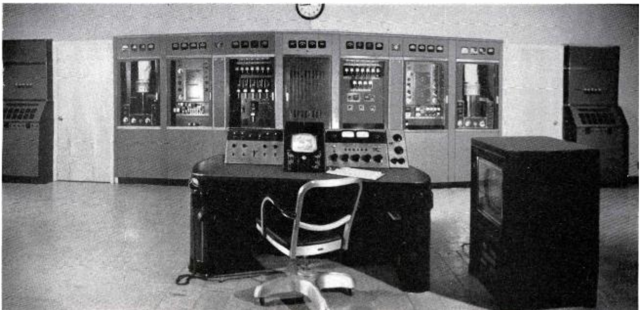
FIG. 2. WISH-TV TT-50AH Transmitter showing in-line arrangement of final amplifiers with driver units. (Distortion in picture is due to use of two negatives.)
