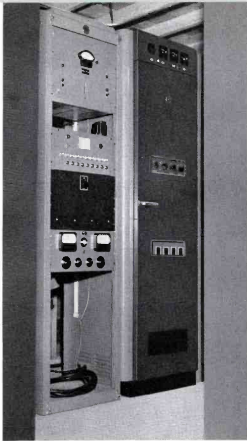
FIG. 17. The KBZY transmitter building houses rack of remote-control equipment and BTA-250M Transmitter.
