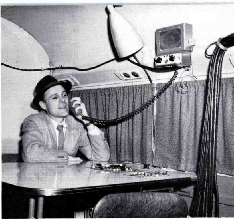
FIG. 52. Alan MacIntyre, Chief Engineer, at director's control of remote unit, using VHF 2-way radio communication system.
