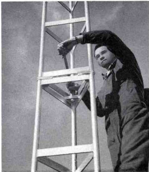
FIG. 5. Two sections of tower are being bolted together. The joint should provide electrical continuity as well as structural strength.
