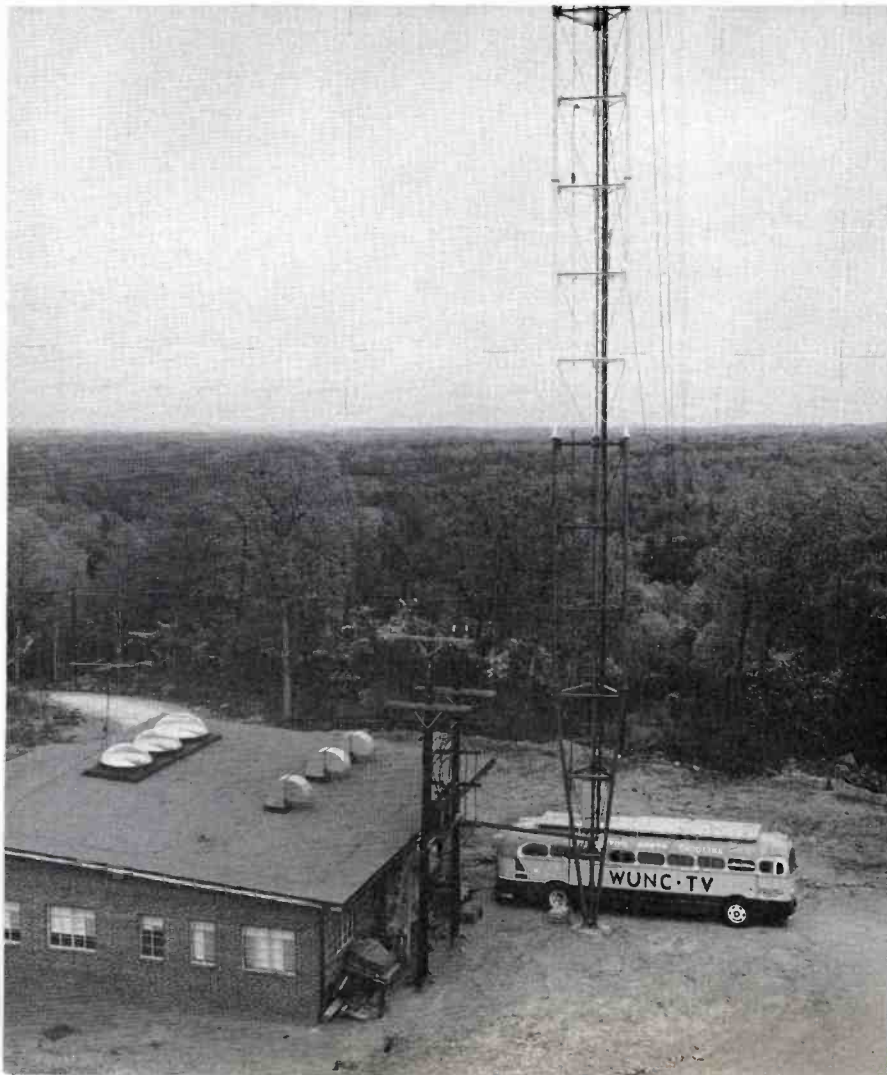
FIG. 36. WUNC-TV transmitter site is approximately eight miles southwest of Chapel Hill, atop Terrell's Mountain, Chatham County. Note plastic "bubbles" in roof, housing microwave dishes.
