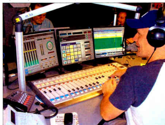
The E-6 in operation in the KUPD Control Room.
