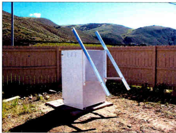
Powder coated aluminum iPowerPV solar shelter with an integrated solar module rack in place.
