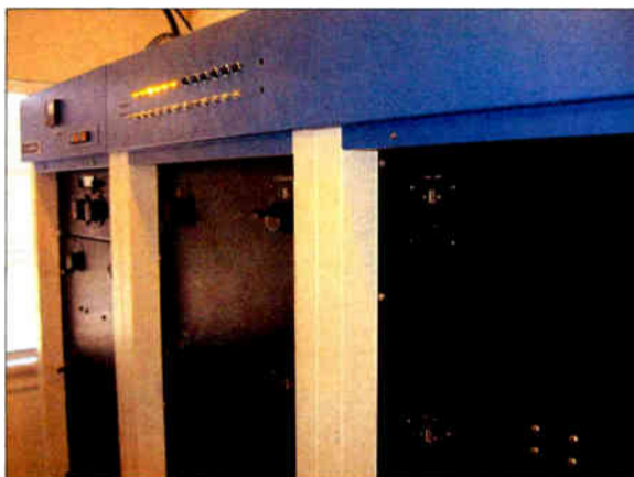
The yellow tally lights show switches set for daytime operation, the dark blue indicates nighttime position.
