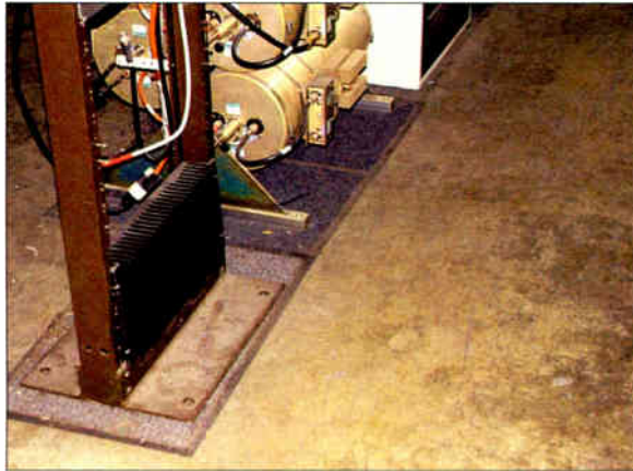
Even a doormat can be used to keep equipment from contacting the floor.
