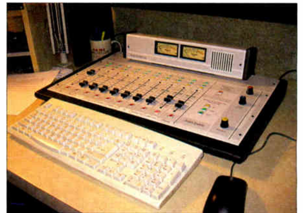
The production room utilizes another ARC-10.
