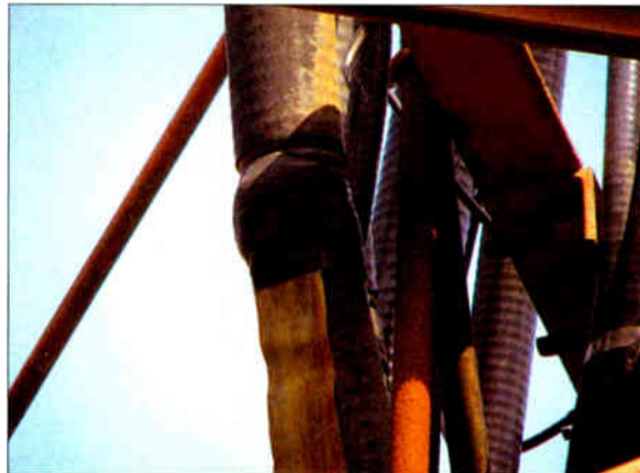
Bonding descending cables to ground.
