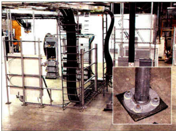
Whenever possible, avoid providing a straight path for strike current.
