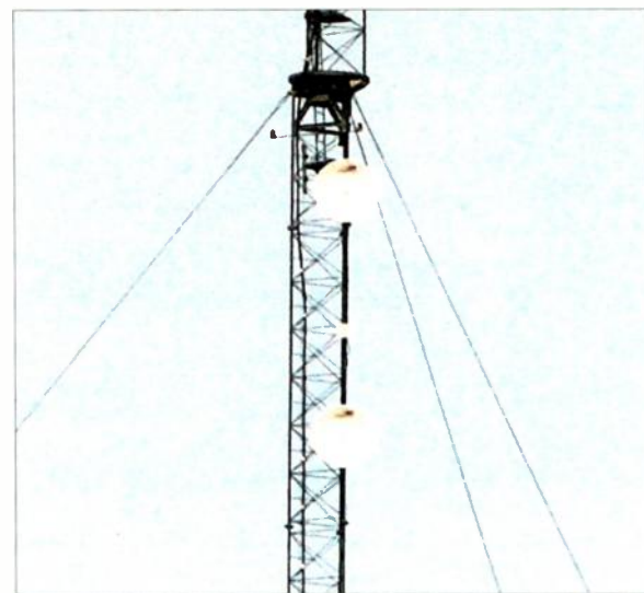
The mounted system. The white box between the antennae is the radio's ODU.
