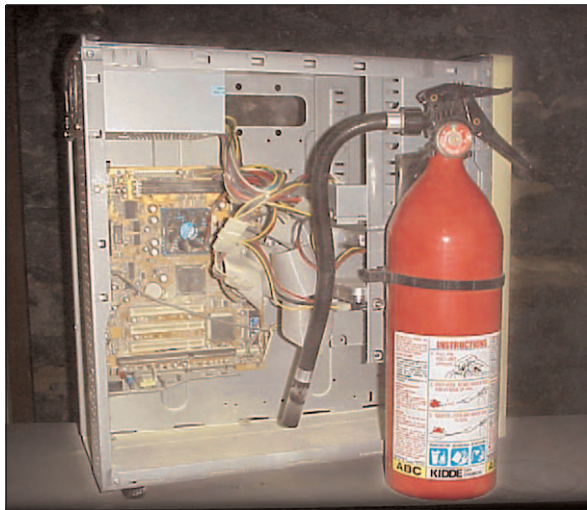
Ruined by a powder type extinguisher
