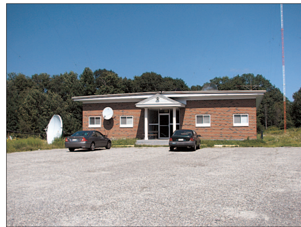
KLOB's studio was completely submerged. Tower #4 is in the background.
