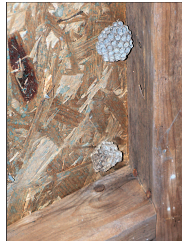
Clean out old bees nest tucked under an exposed roof soffit.
