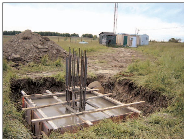
The Monopole base partially completed.
