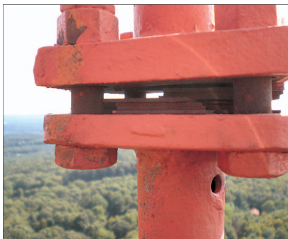
The Second Flange with Shims
