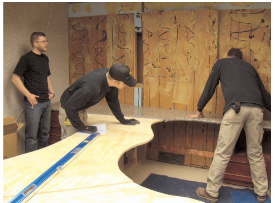
The New Countertop
