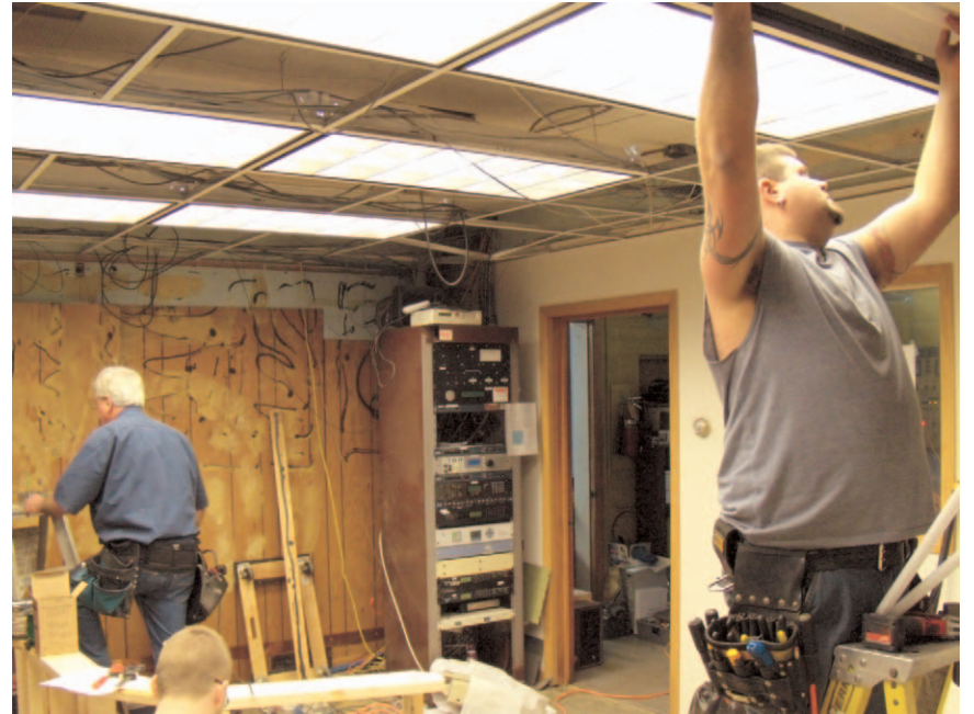
New Lighting Being Installed
