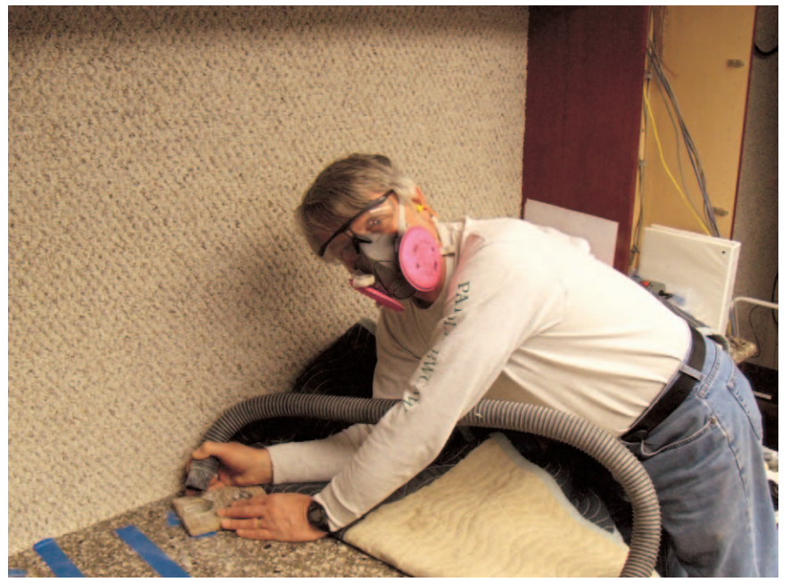
Cutting Holes in the Counter Top
