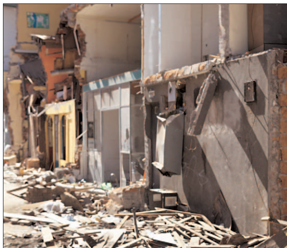
Buildings were reduced to piles of rubble.
