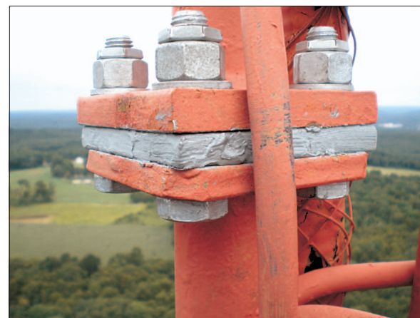
The Proper Spacer Bolted in Place
