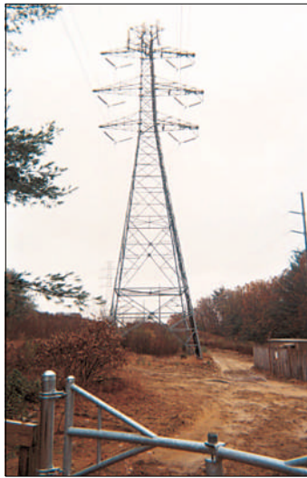
High tension wires on site. The power tower had to be detuned.
