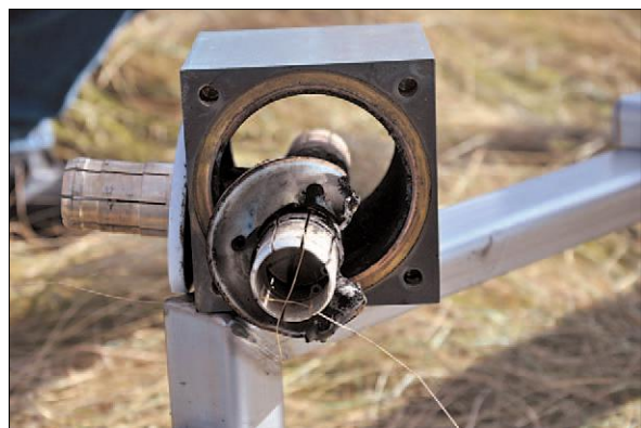
One of several damaged parts found on the antenna.
