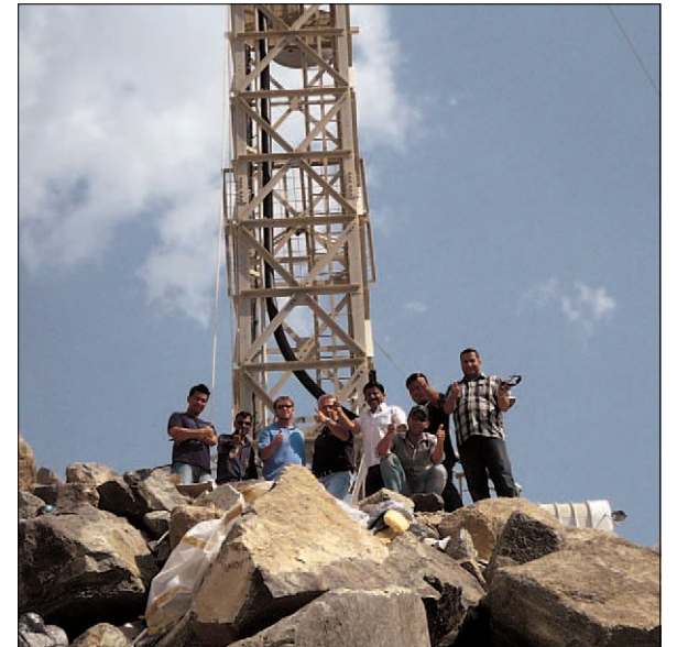
Thumbs up by the crew after a successful installation of an antenna and combiner system in Dubai. Matt Smith and Martyn Gregory are in the center.
