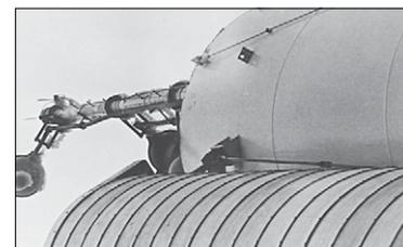
Looking up from the 110th floor roof level at the temporary FM mast atop the west base. This shows some ice buildup on the antenna radome.
