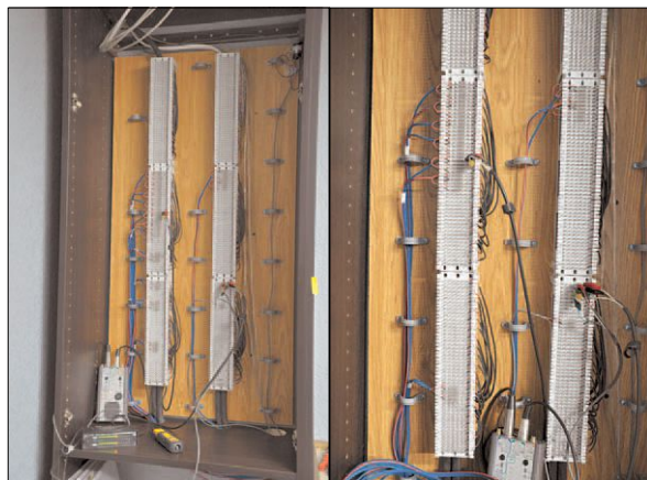
Partial Wiring in Place
