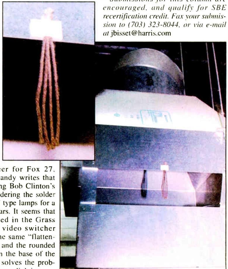
Figure 3: Here's a simple, effective way to ensure that positive outside air pressure is not defeating your cooling system.
