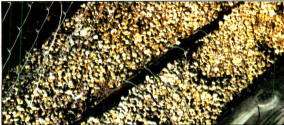
Figure 6: Ground radials are shown attached to the copper ground screen at the base of the tower.
