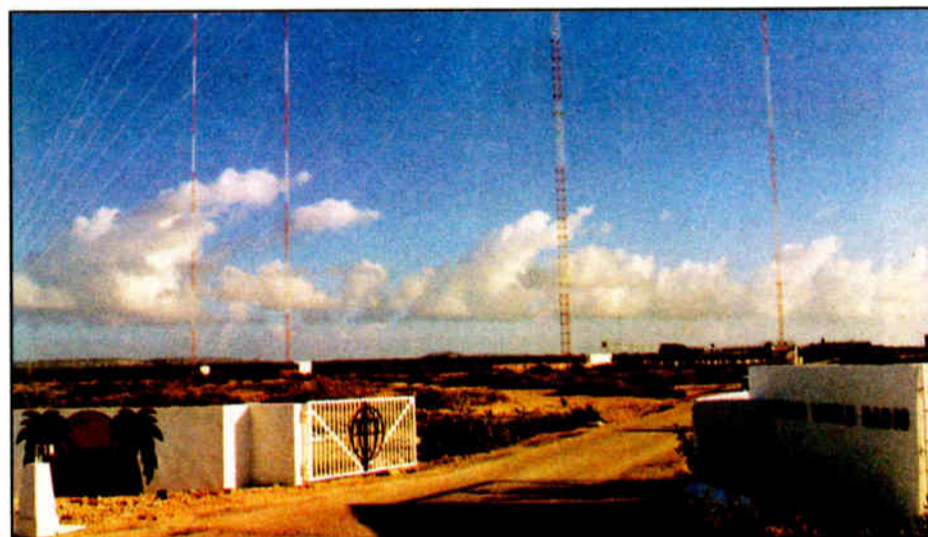
This five-tower array belongs to Trans World Radio in Bonaire in the Netherlands Antilles. The 500 kW station broadcasts at 800 kHz.
