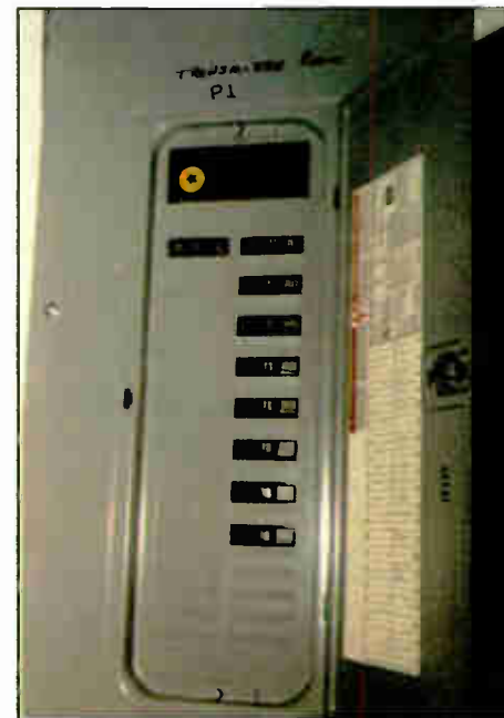
Fig. 2: Be sure that all hard-drive computers are on the same phase.
