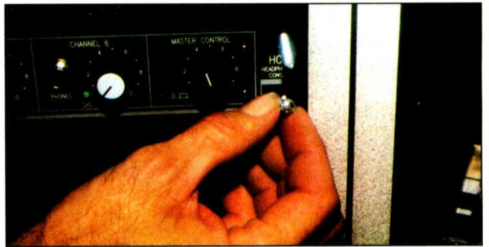
Fig. 2: A modified bolt can support equipment in a rack
