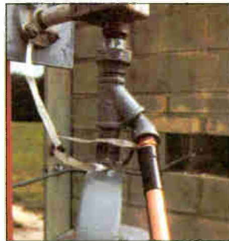
Fig. 3: Ensure that grounds are connected properly
