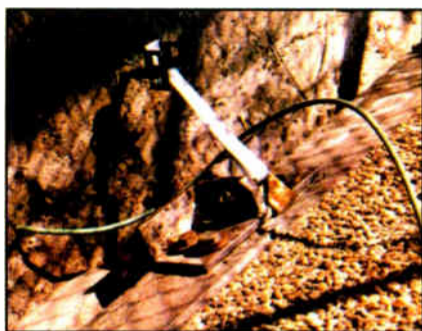
Fig. 4: Make sure that building grounds are intact
