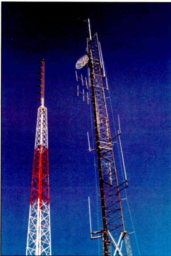
Shown are two skirted towers on Mt. Scott in Portland, Ore. The left tower supports an FM antenna and serves as an AM radiator. The wireless tower on the right also supports a one-bay FM aux antenna.
