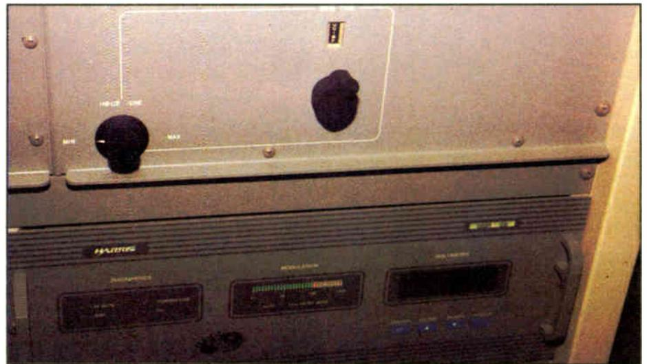
Fig. 2: Keep a spare fan for your exciter and verify a proper match into the transmitter.
