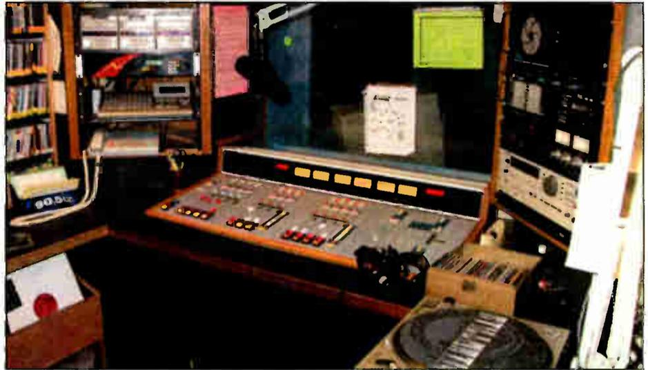
**KSJS(FM)** has a new **Wheatstone D-5000** audio digital console and **Wiremax Studio Interface System**.
