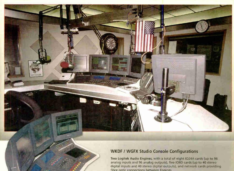
fibre optic connections between Engines
