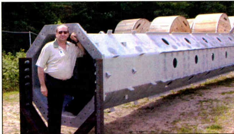
John Lyons pauses during inspection of the upper UHF steel tower spine as shipped from ERI, before Dielectric mounted the antennas, transmission lines, power dividers and radome.
