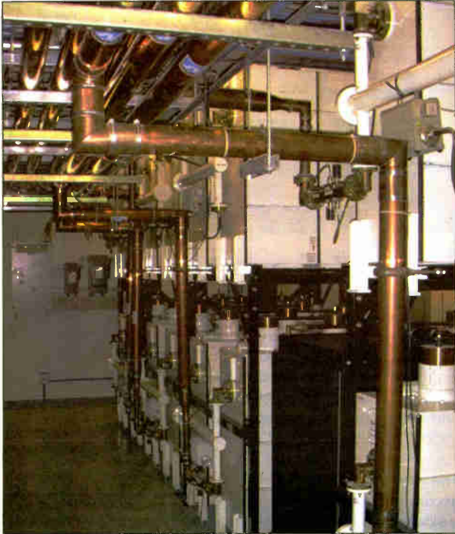
Shown is part of the input side of the Shively FM combiner system. The short black rack is the Harris Recon Monitor System cabinet.
