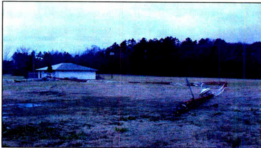
The fallen tower is shown near the transmitter building.
