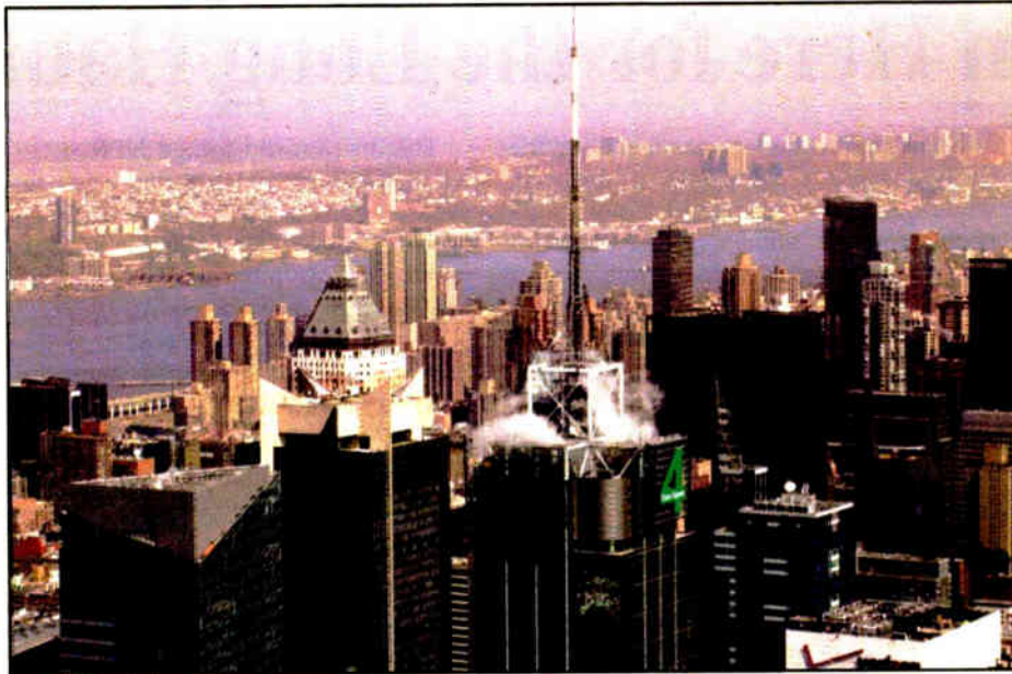
The new structure is a notable presence in midtown Manhattan. Times Square is on the right.
