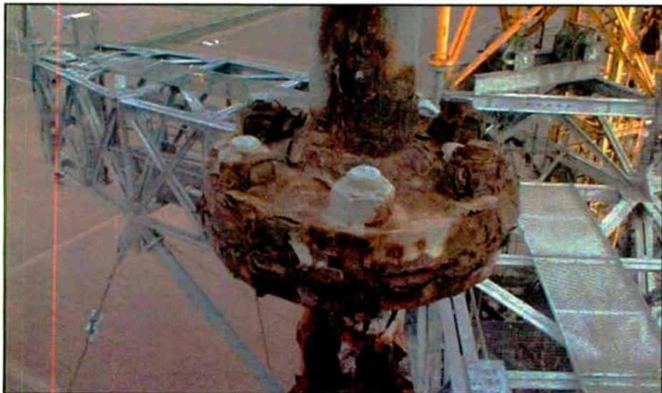
Fig. 1: Rust can form anywhere on a tower.
