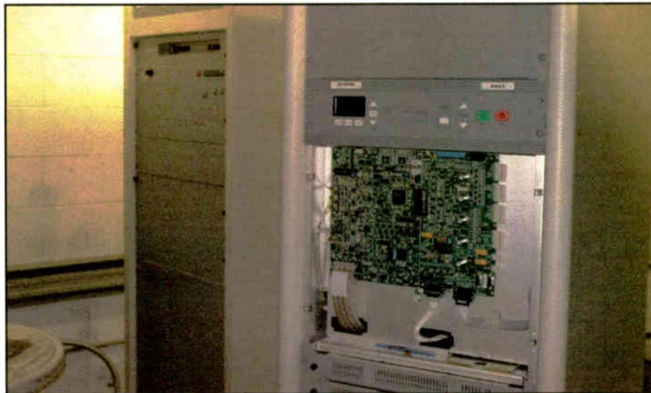
Fig. 3: On most solid-state transmitters, critical backup settings are kept 'alive' with a backup battery. Make sure it's fresh.
