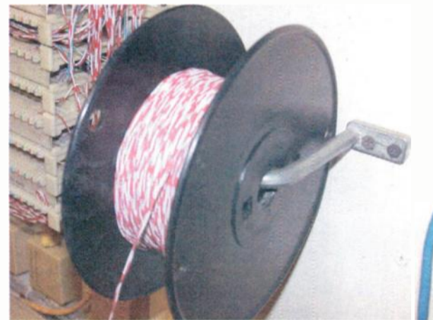
Fig. 3: A D-ring efficiently holds a spool of cross-connect wire.
