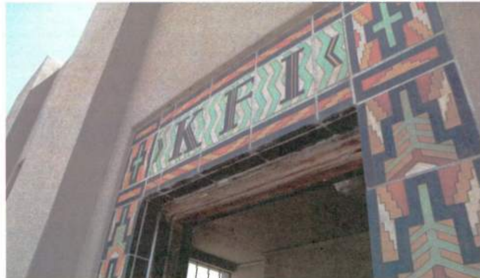
Art Deco tilework around the front door at KFI.
