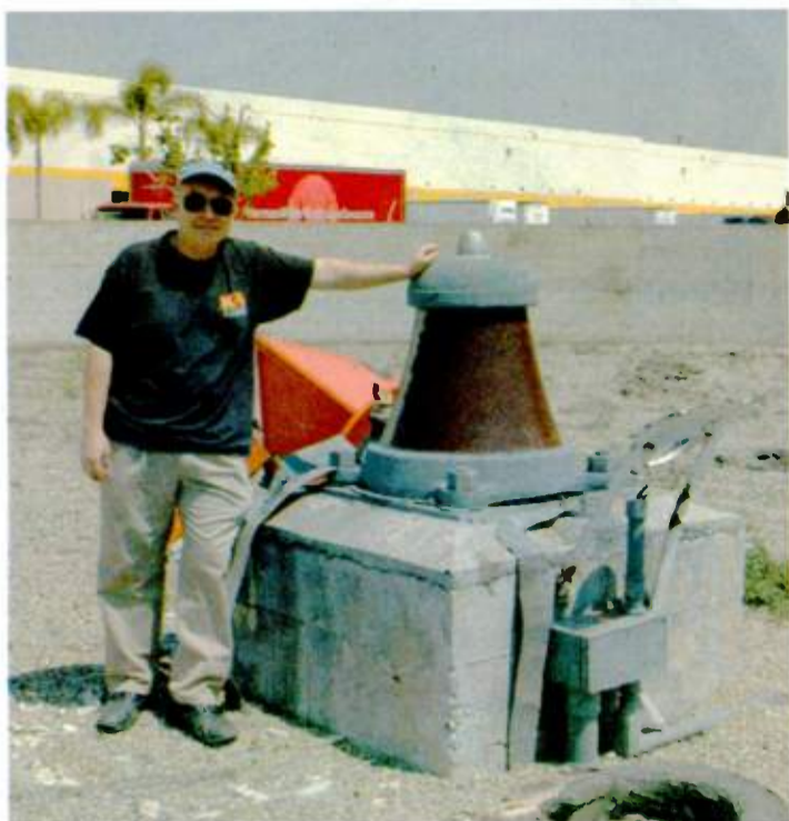
KFI Chief Engineer Tony Dinkel with the base of the tower after the plane crash.
