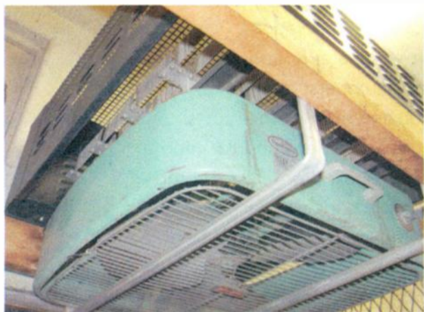
Fig. 1: Add a box fan to improve dummy-load cooling.
