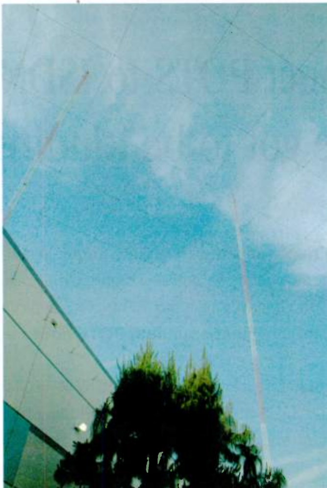
KTNO/KTLK's towers rise above the industrial park. A screen of wires extends over the parking lot between warehouse buildings and serves as part of the grounding system; it ties into chicken wire that lines the walls and roofs of the buildings.
