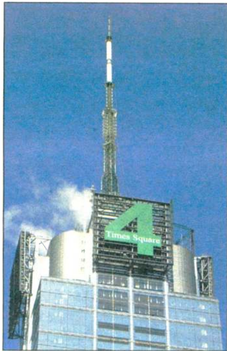
Fig. 4: The 4 Times Square building showing the antenna mast with master antennas for FM radio and VHF and UHF TV broadcasting.
