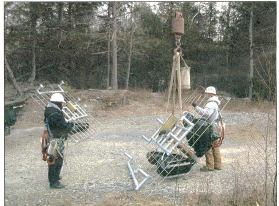
Fig. 7: Assembled Panel About to be Lifted to Tower
