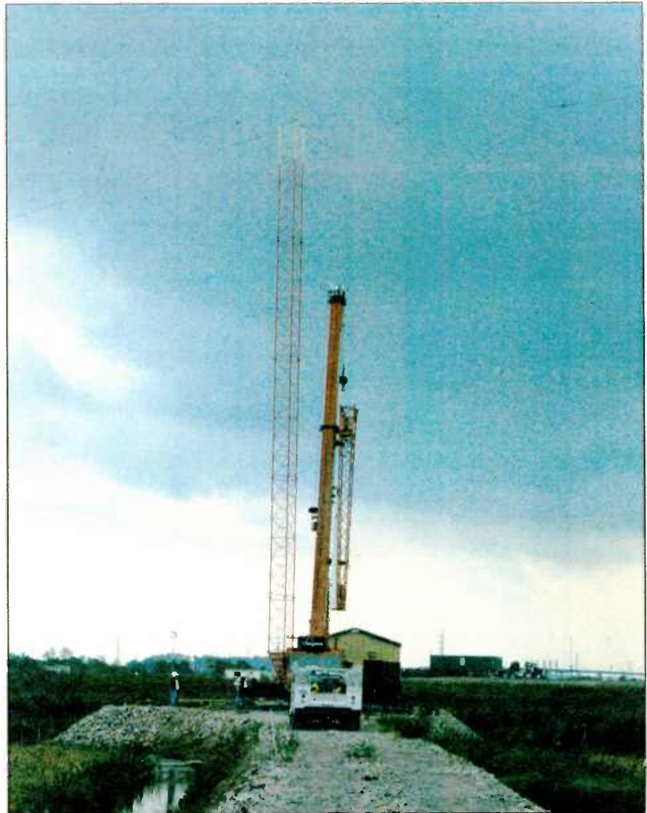
The first 100 feet of Tower 2 stands as the crane is lowered.
