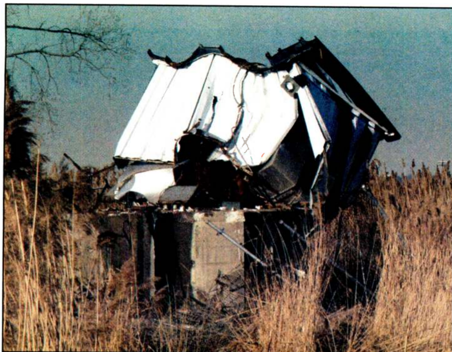
Lyndhurst Tuning House One was hit by guy wires. The other two tuning houses survived without a scratch.
