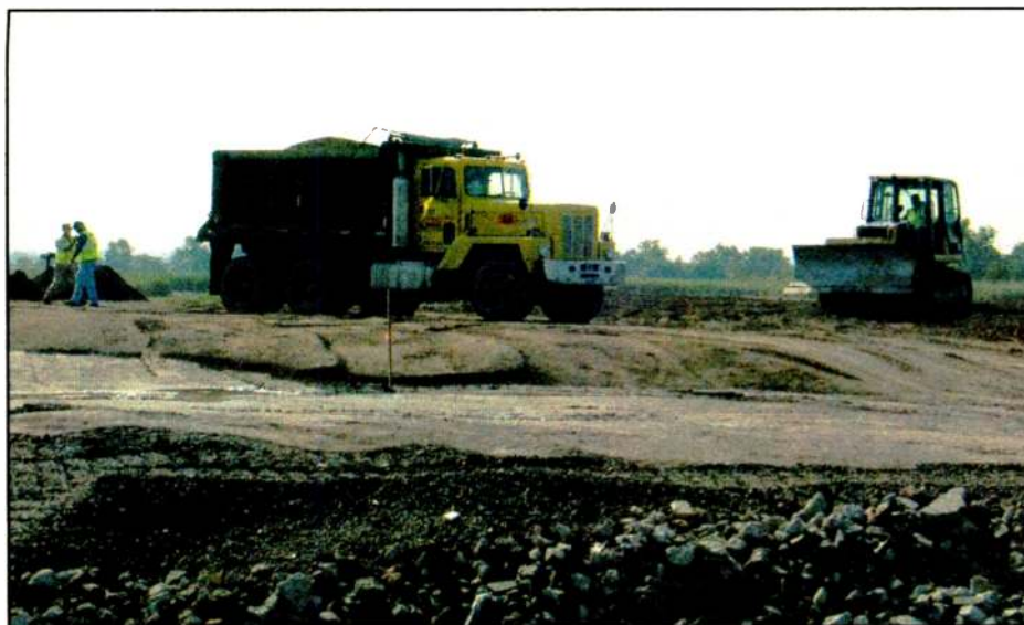
Dump trucks bringing fill material to the WOR property.
