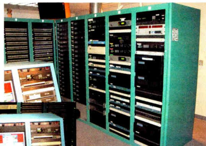
Master Control Room, where Stantron Pioneer racks house network operations gear, such as uplink gear, encoders and digital automation equipment.
