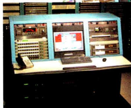
The Frontier console system houses a computer workstation that controls Dial Global's satellite receivers.
