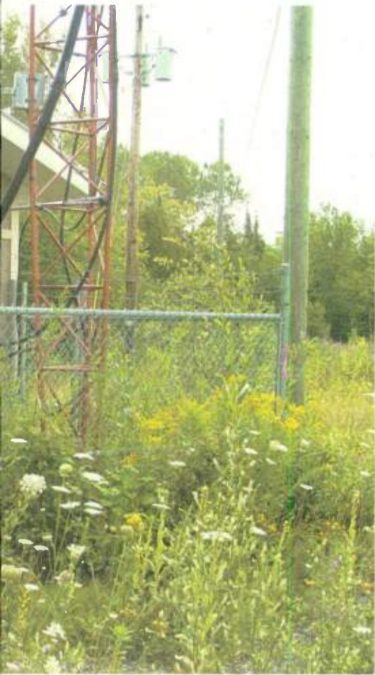
building are grounded properly.
