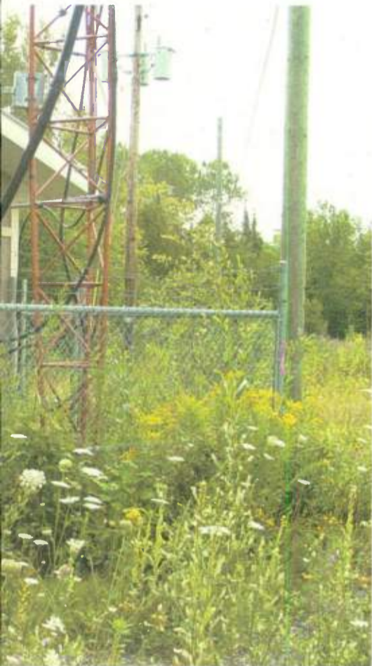
building are grounded properly.
