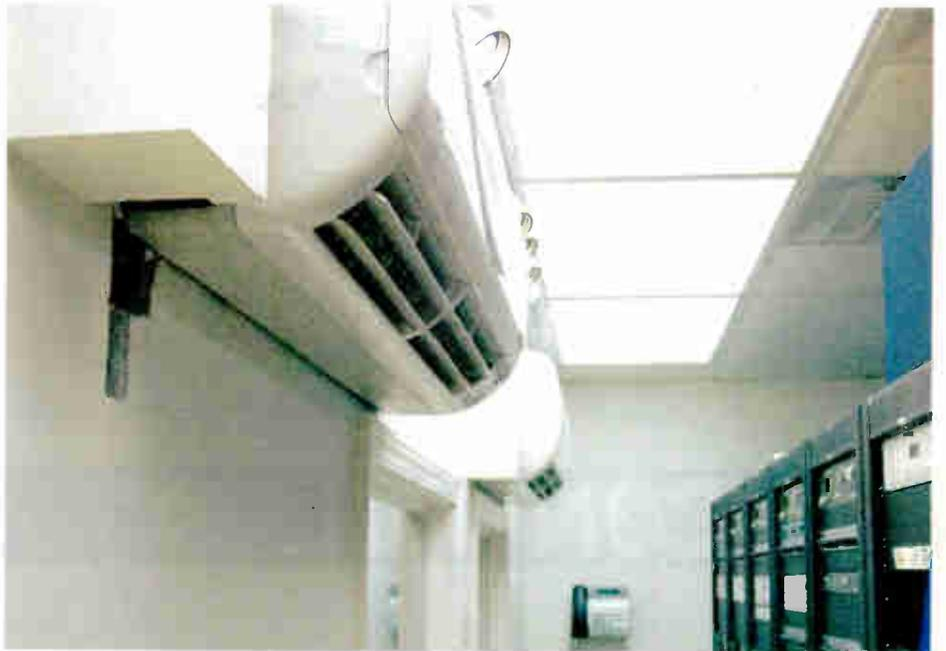
Fig. 2: Wall-mounted air conditioners are an excellent cooling choice for rack rooms.
