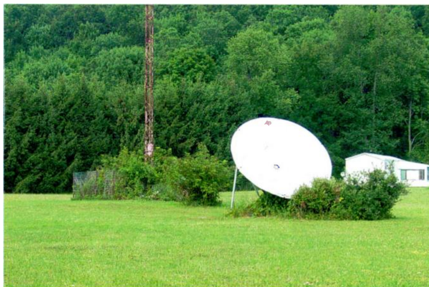
Fig. 6: Avoid a fine and deter vandals. Trim vegetation from your tower, building and satellite dish.
