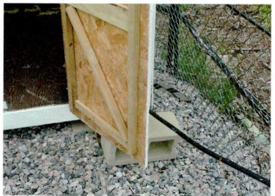
Fig. 2: When the door swung open, it shook the transmission line.
