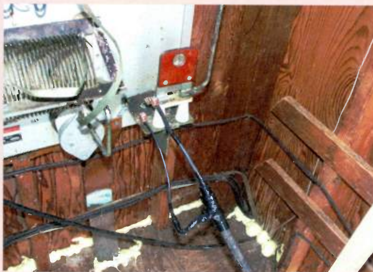
Fig. 3: The repair to the transmission line ensured no more shorting.
