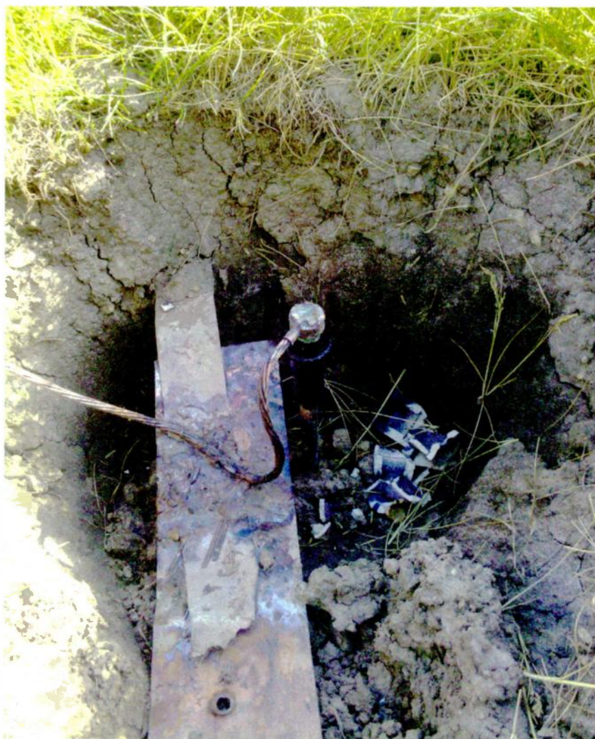
Fig. 6: Seven-strand copper wire can be used as a pigtail.
